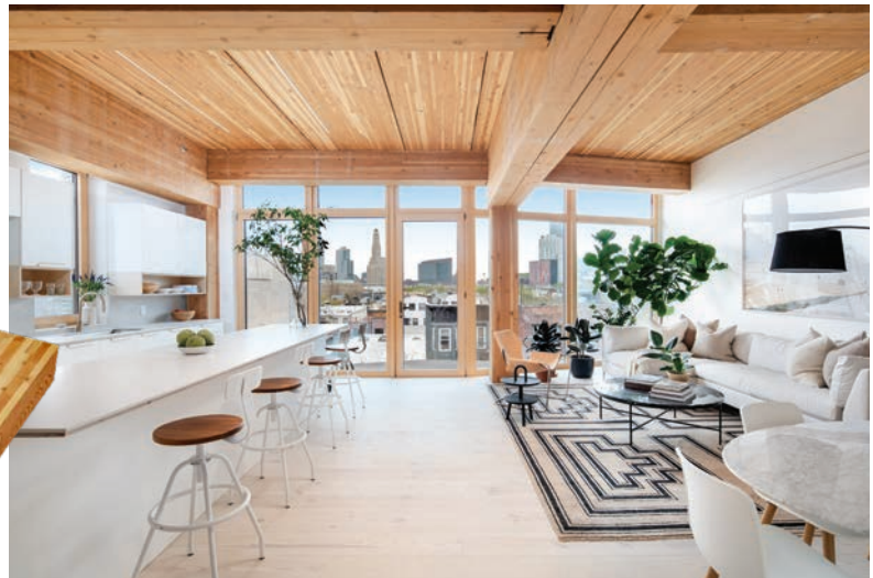
Glulam columns and beams and GLT ceilings at Timber House in Brooklyn, NY Mesh Architectures / Silman Structural Solutions
