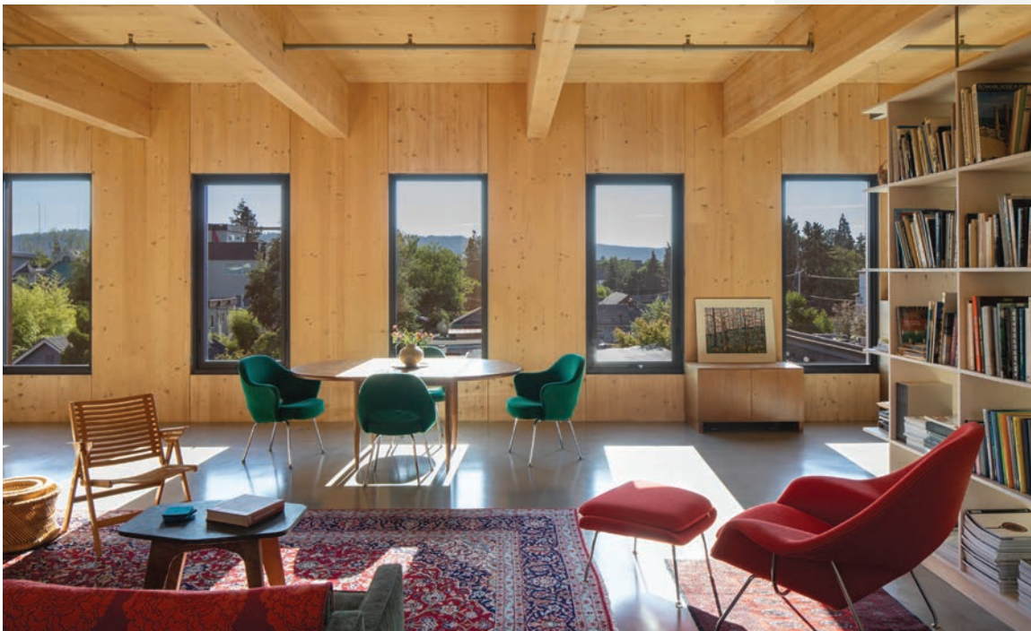
CLT walls and ceiling at Mississippi Workshop in Portland, OR Waechter Architecture / KPFF
