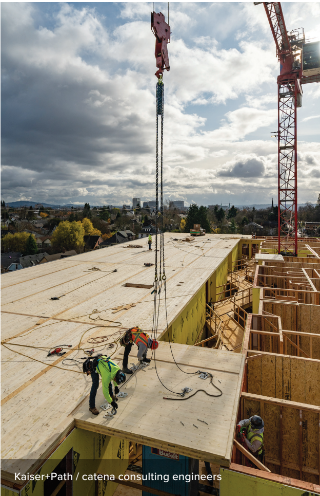
Panel-to-panel connections with splines at The Canyons in Portland, OR
