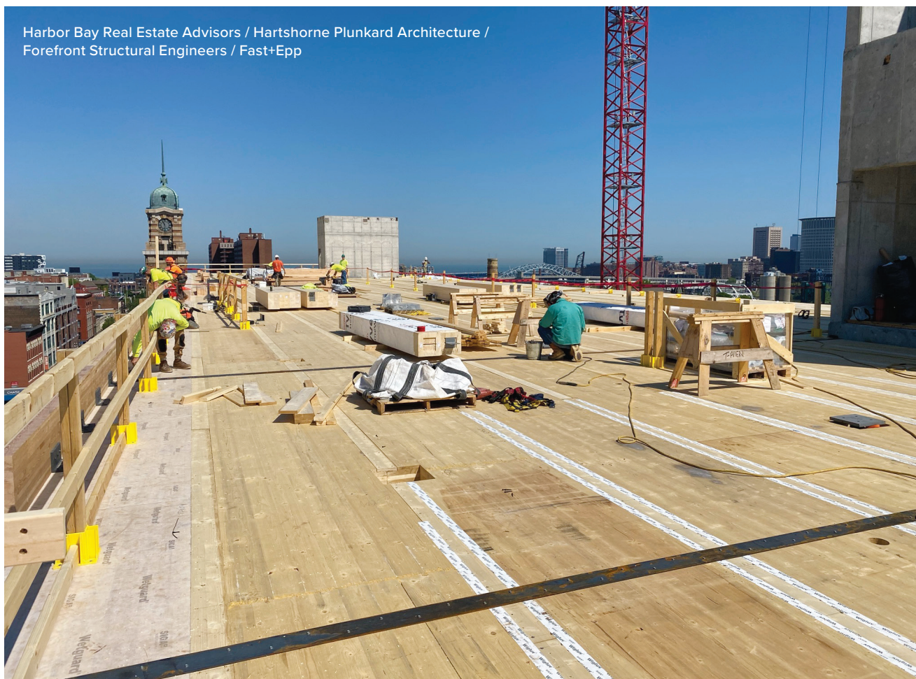
Installing spline tape at INTRO in Cleveland, OH
