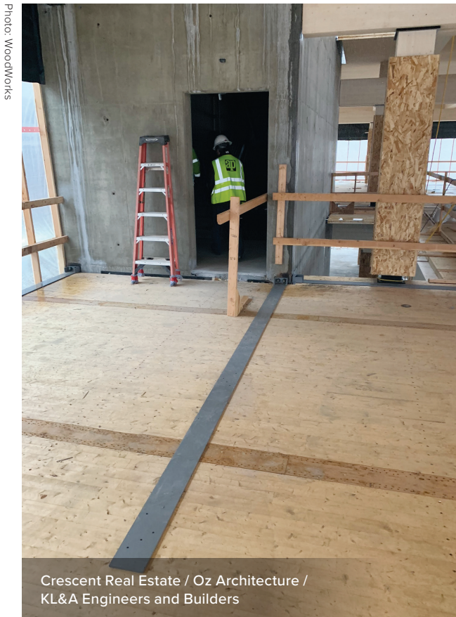
Collector strap from CLT diaphragm to core walls at Platte Fifteen in Denver, CO
