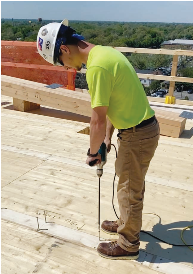
The hammer setting on rotary drill equipment is not recommended for installing threaded fasteners in mass timber. Not all fasteners are the same and the fastener manufacturer should be consulted for installation instructions.
