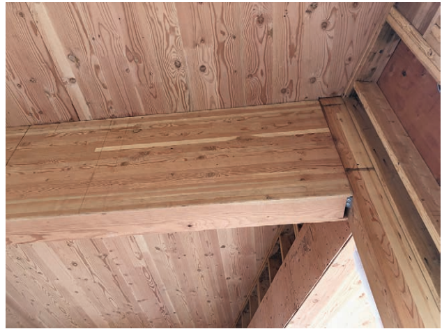
The concealed hanger in this glulam beam-to-column connection is not fully seated.
