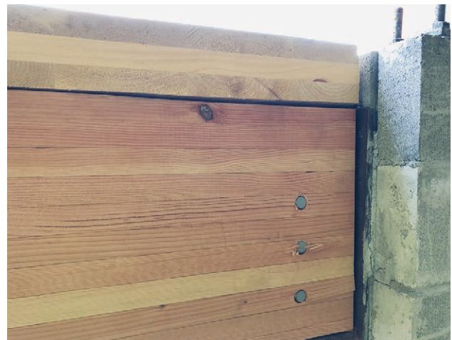
The fit-up of this glulam beam against the masonry wall created a gap where the CLT panel bears on the beam. Long bearing seats and field-drilled holes for the pins allowed for field adjustability of the beam-to-wall connection.
