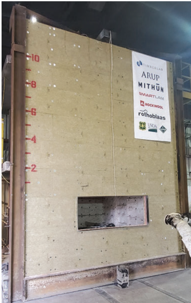
FIGURE 7: Completed wall setup prior to testing
