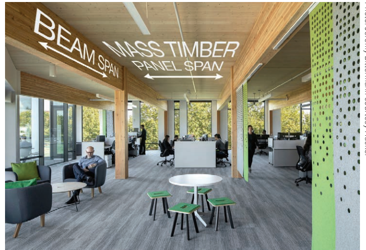
One-way mass timber post-and-beam framing scheme
