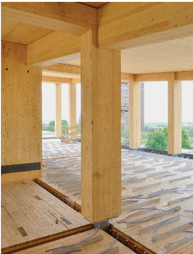
Electrical conduit placed above mass timber floor panel prior to topping slab pour at the John W. Olver Design Building at UMass Amherst / Leers Weinzapfel Associates
