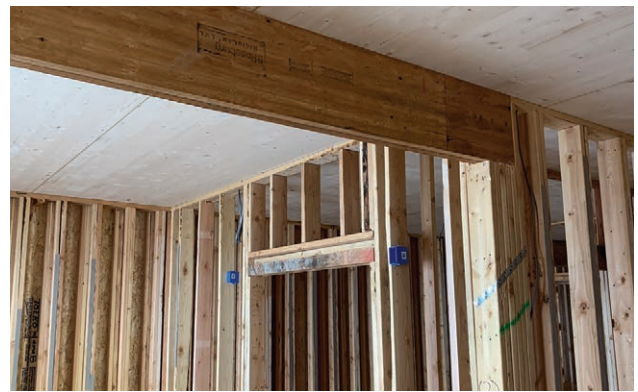
Mass timber floor panel supported on light-frame bearing wall and wood beam within multi-family dwelling unit
