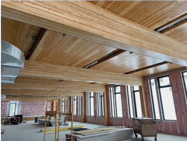
Gapped mass timber panels with electrical routed in chases at the PAE Living Building
