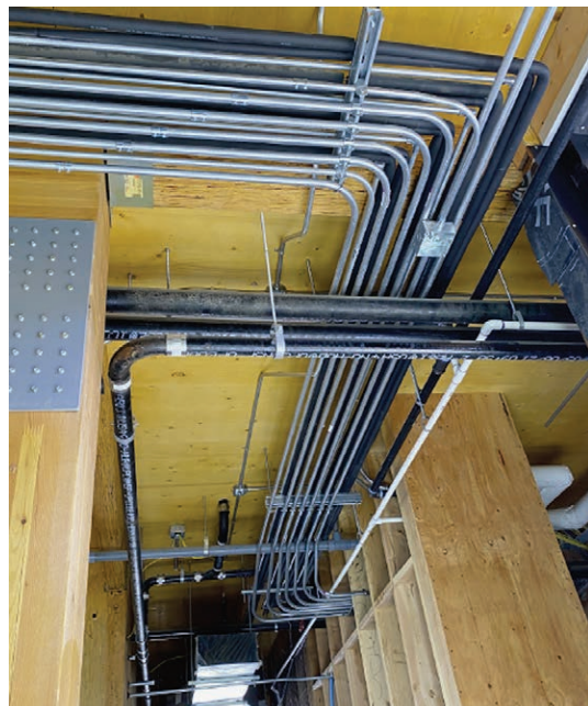
Exposed MEPF at Sonrisa / 19six Architects
