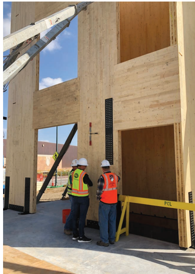
CLT shear walls at the University of Denver Burwell Center
