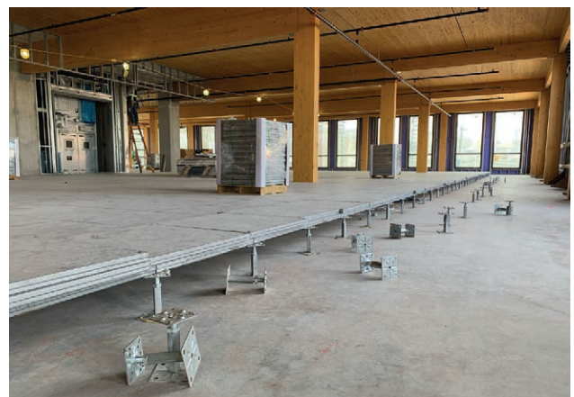
Raised access floor being installed in a mass timber building
