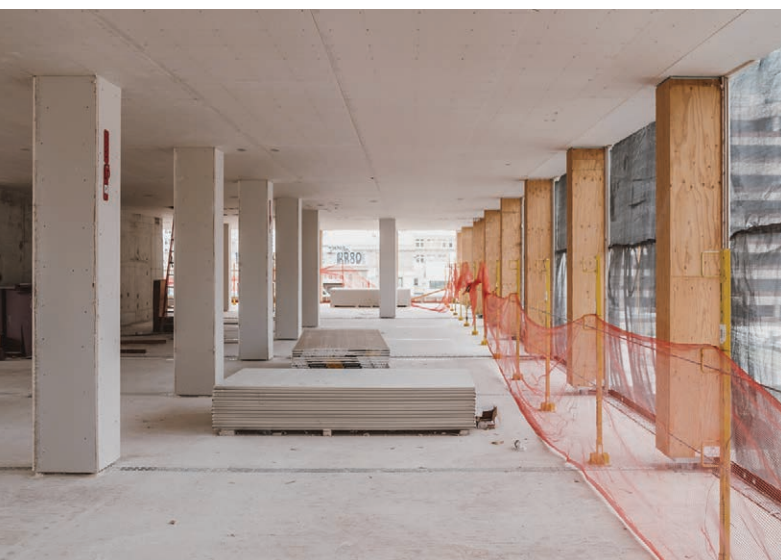
GWB installation nearly complete at 1510 Webster in Oakland, CA
