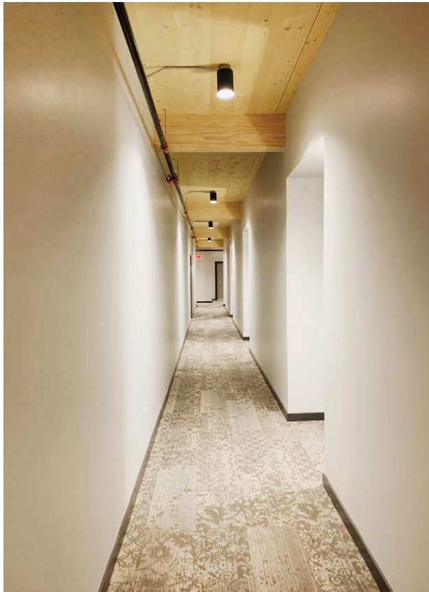
CLT floor/ceiling panels in a corridor with intermediate beams at Timber Lofts / Engberg Anderson Architects
