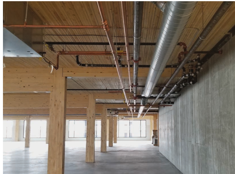
Shallower beams adjacent to a core accommodate larger MEPF lines at T3 Minneapolis / MGA | Michael Green Architecture / DLR Group / Magnusson Klemencic Associates / StructureCraft
