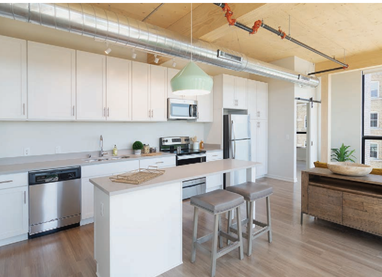
Ductwork and sprinkler lines hung below beams at Timber Lofts / Engberg Anderson Architects / Pierce Engineers
