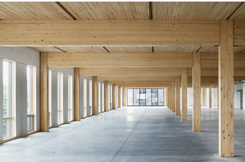
Gaps between panels create space for sprinkler lines at 111 East Grand / Neumann Monson Architects / Raker Rhodes Engineering / StructureCraft
