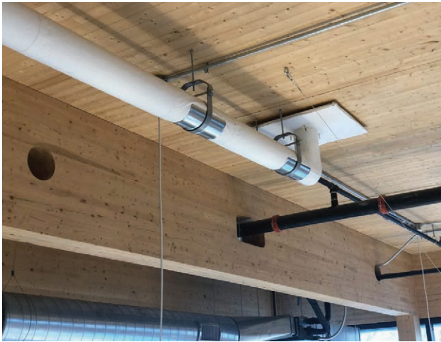
Precut holes in a glulam beam for MEPF routing
