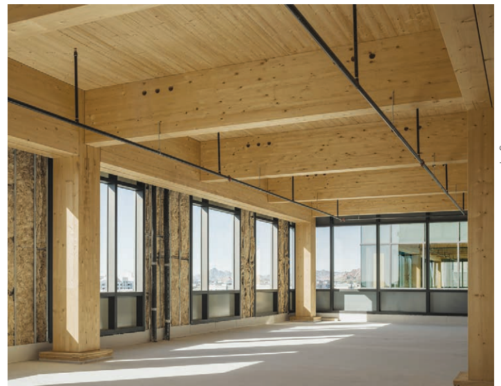
Two-way beam system at The Beam on Farmer / RSP / PK Associates
