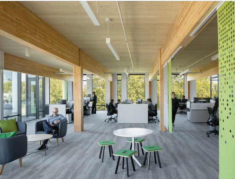
One-way beam system at the First Tech Federal Credit Union / Hacker / Kramer Gehlen & Associates
