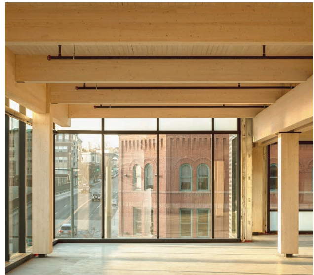
Stacked beam system at Platte Fifteen / OZ Architecture / KL&A Engineers and Builders
