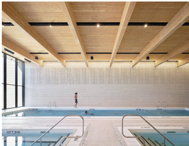
In the aquatic center of the San Antonio Spurs' Victory Capital Performance Center, larger gaps between panels provide enough space for electrical and lighting / ZGF / Arup
