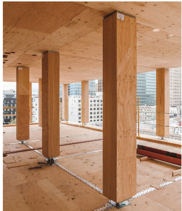
Point-supported mass timber panels at 1510 Webster / oWOW / DCI Engineers
