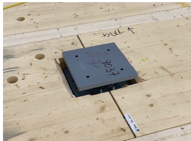
In this photo, the column connection and diaphragm splines would not have code-required special inspections. However, if additional fasteners were applied to the spline at spacings closer than 4 inches on center, special inspection would be required.
