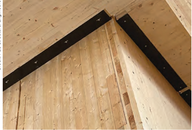
CLT floor panel supported on CLT shaft wall by steel ledger angle
