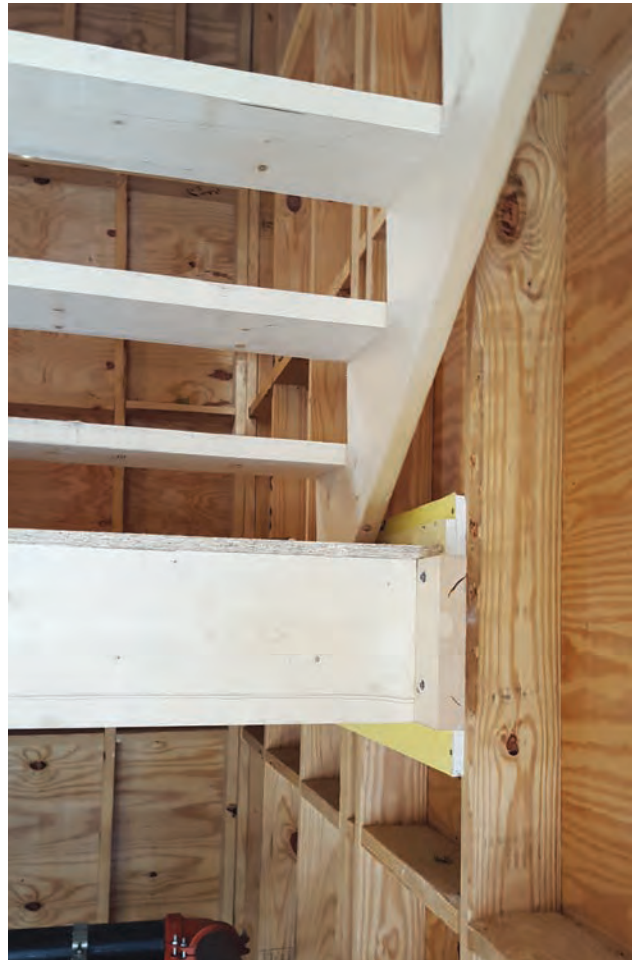
Stair landing framing attached to shaft wall through two layers of gypsum prior to landing beam hanger installation
