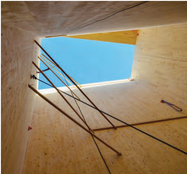
CLT shaft walls at the John W. Olver Design Building at the University of Massachusetts (UMass – Amherst)
