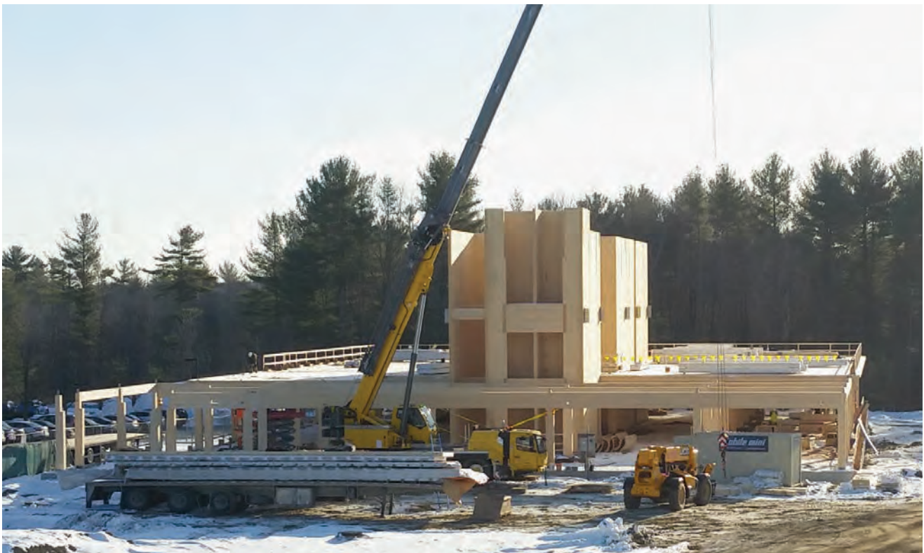
Mass timber shaft walls at 90 Arboretum Drive, a three-story office building in Newington, NH
