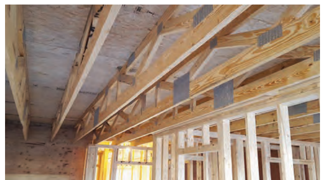
Example of a fire partition wall
