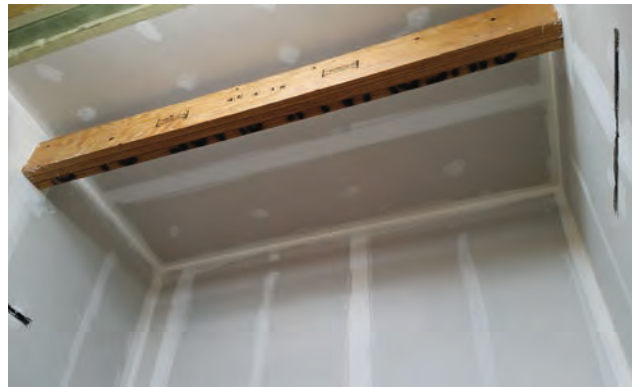
Wood-frame elevator hoist beam
