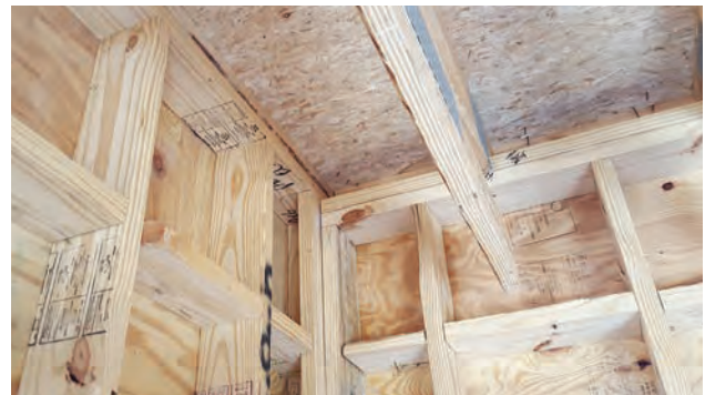
Example of fire barrier wall continuity, extending to underside of floor/roof sheathing above
