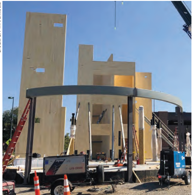
Mass timber shaft walls at the University of Denver's Burwell Center for Career Achievement
