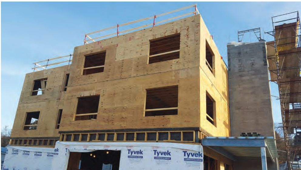
Masonry shaft wall in a wood-frame building
