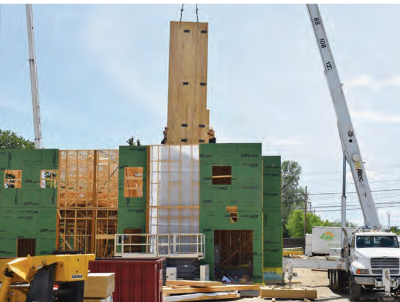
CLT shaft wall installation at Wessex Woods, an affordable housing project in Portland, ME
