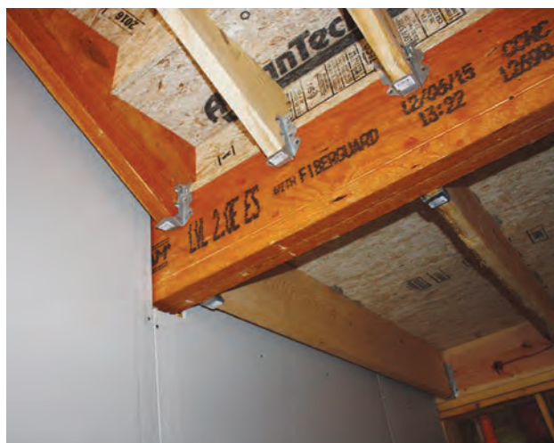
Stair landing beam shaft wall structural penetration prior to firestop system installation
