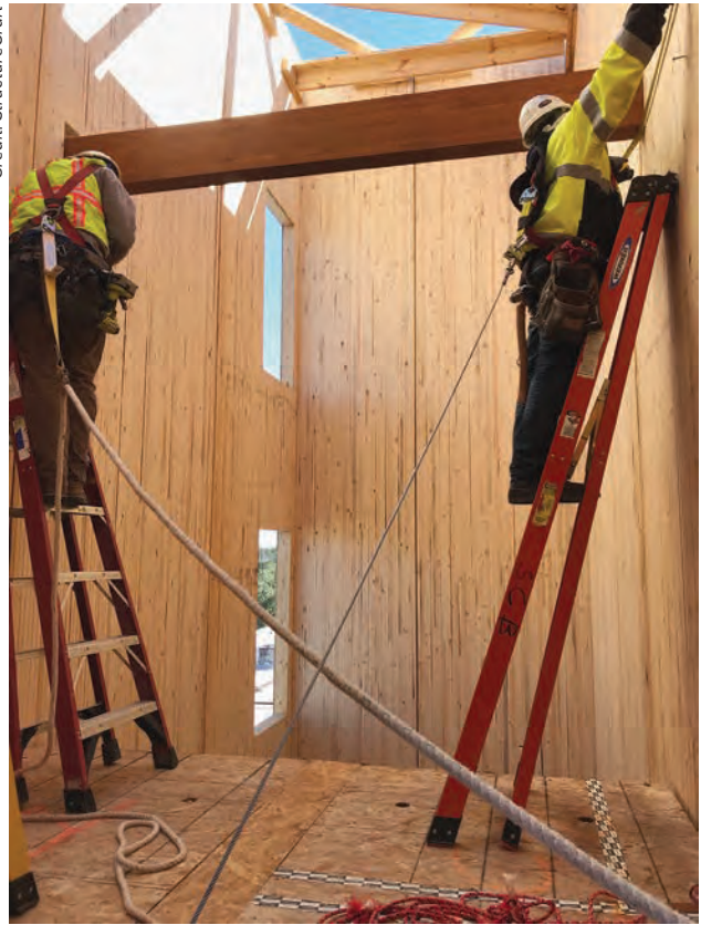
DLT shaft walls at the Magdalena Hotel in Austin, TX
