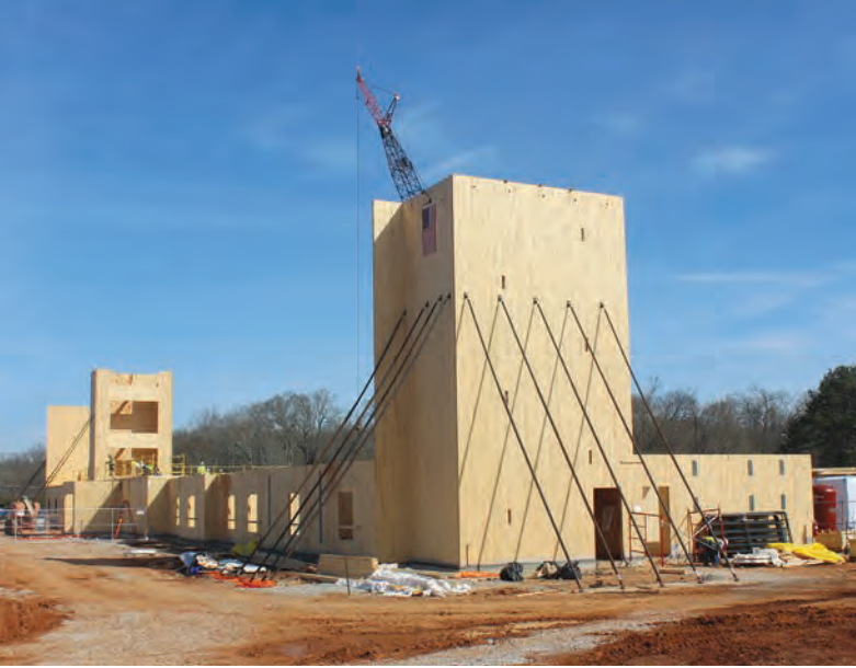
At the Candlewood Suites hotel at Redstone Arsenal, each of the shaft walls was a single, 37.5-foot-long CLT panel.
