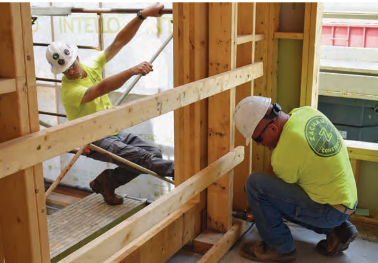
CLT shaft wall installation at Wessex Woods
