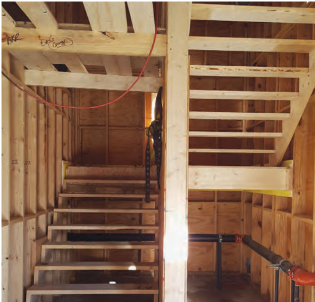
Stair shaft at exterior wall
