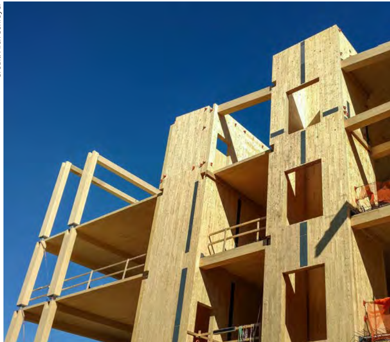
CLT shaft walls doubled as shear walls at the John W. Olver Design Building, providing lateral load (seismic and wind) resistance.
