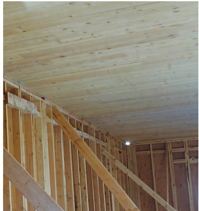
Mass timber floor panel bearing on light wood-frame shaft wall
