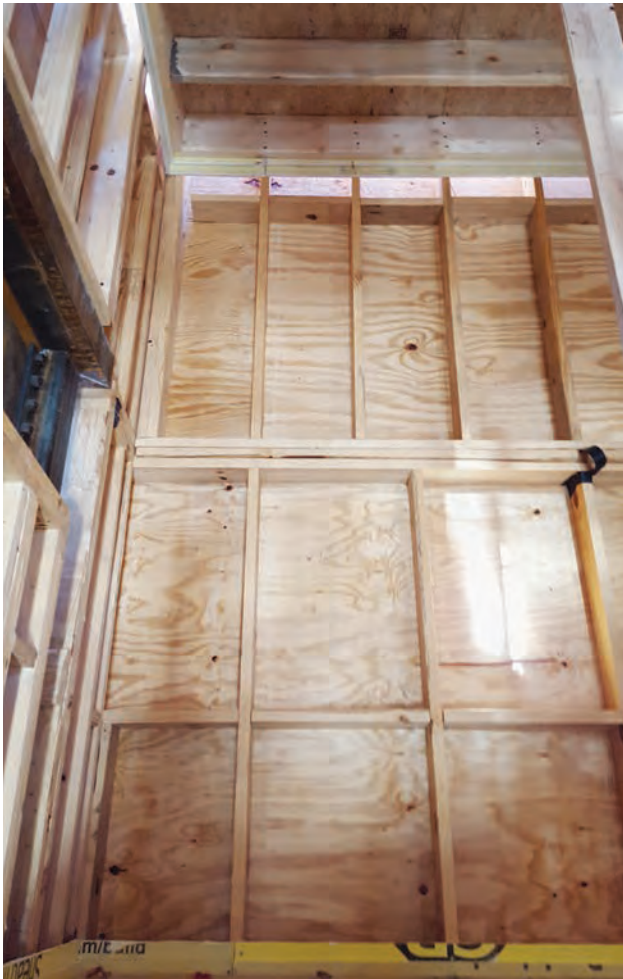
Stair shaft wall stud joints at exterior wall
