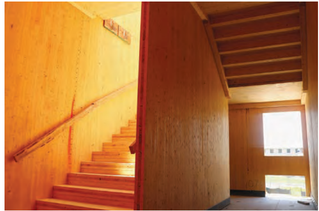
CLT was used for stair framing and shaft walls at the Candlewood Suites Hotel at Redstone Arsenal, AL
