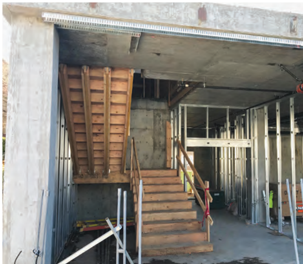
Example of wood stair framing below the podium in a mid-rise project
