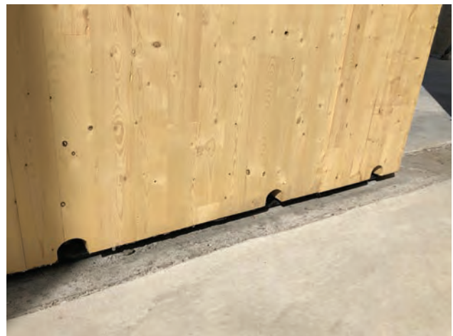
CLT shaft wall base anchorage inspection holes at the Burwell Center for Career Achievement
