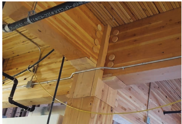
Exposed connections protected with wood coverings
