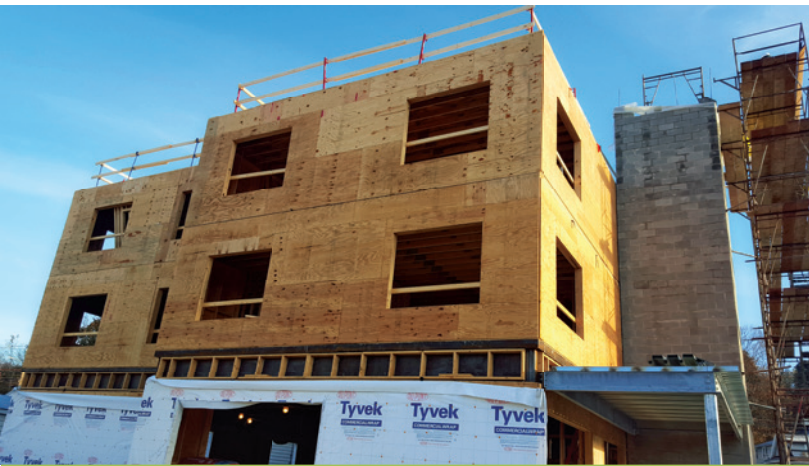
Masonry shaft wall in wood-frame building
