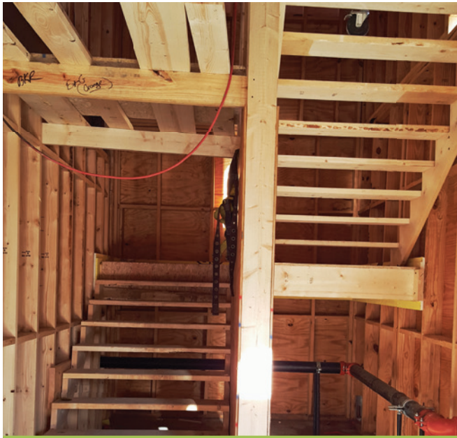
Stair shaft at exterior wall
