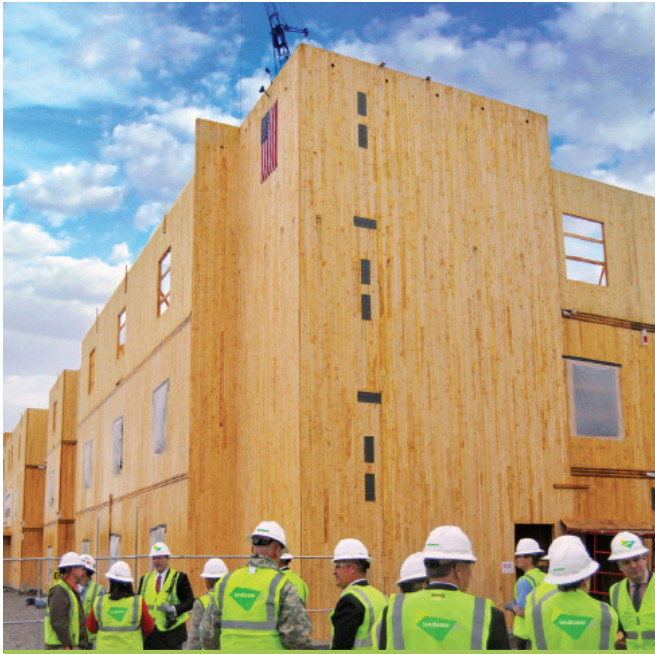
The four-story Candlewood Suites® at Redstone Arsenal, Alabama, is made entirely from CLT – including the shaft walls.
