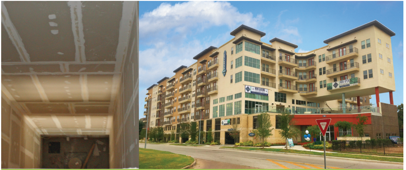
Wood shaft walls can reduce costs and shorten the construction schedule.
