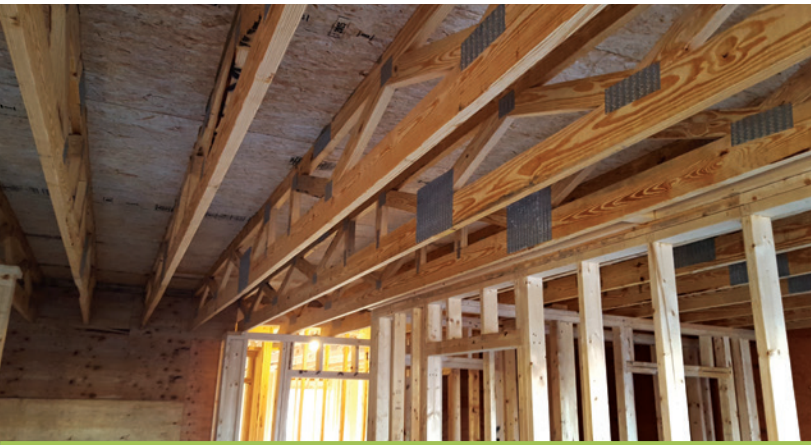
Example fire partition wall
