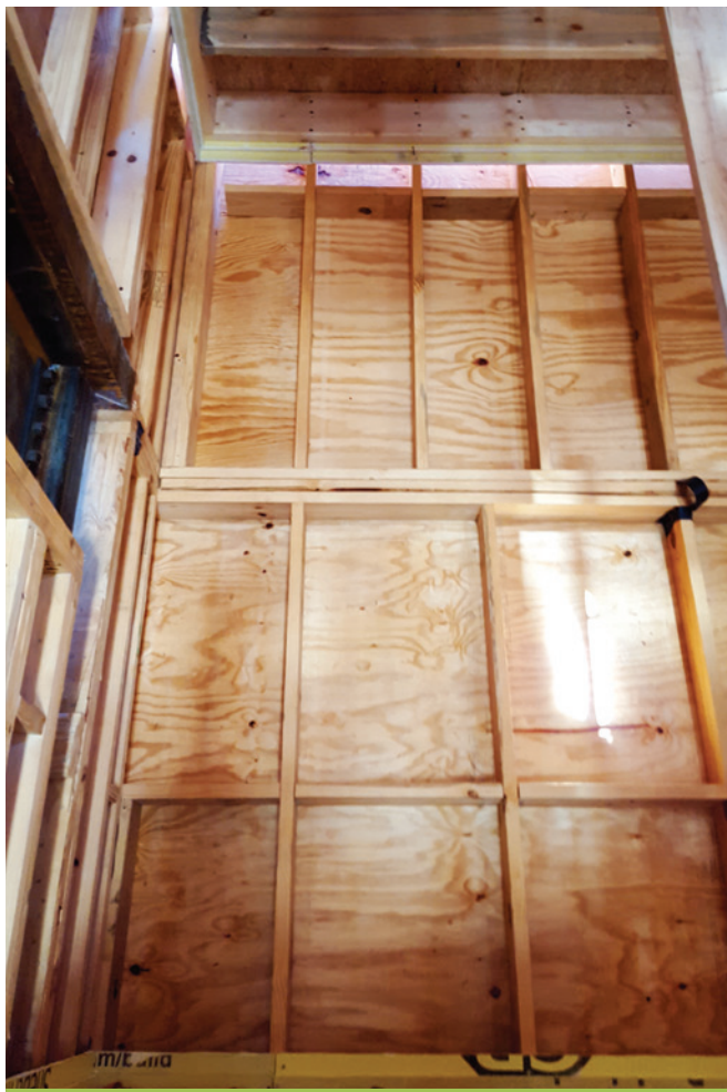
Stair shaft wall stud joints at exterior wall
