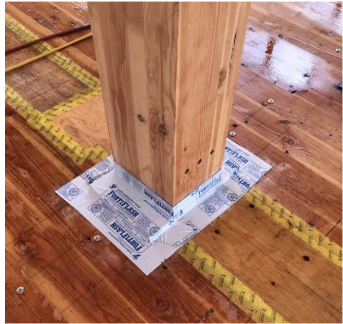
Figure 7: Example of construction moisture management technique
