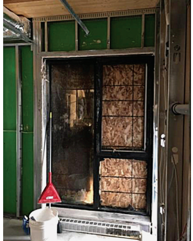
Figure 11: Fire damage in the Arbora complex in Montreal, QC
