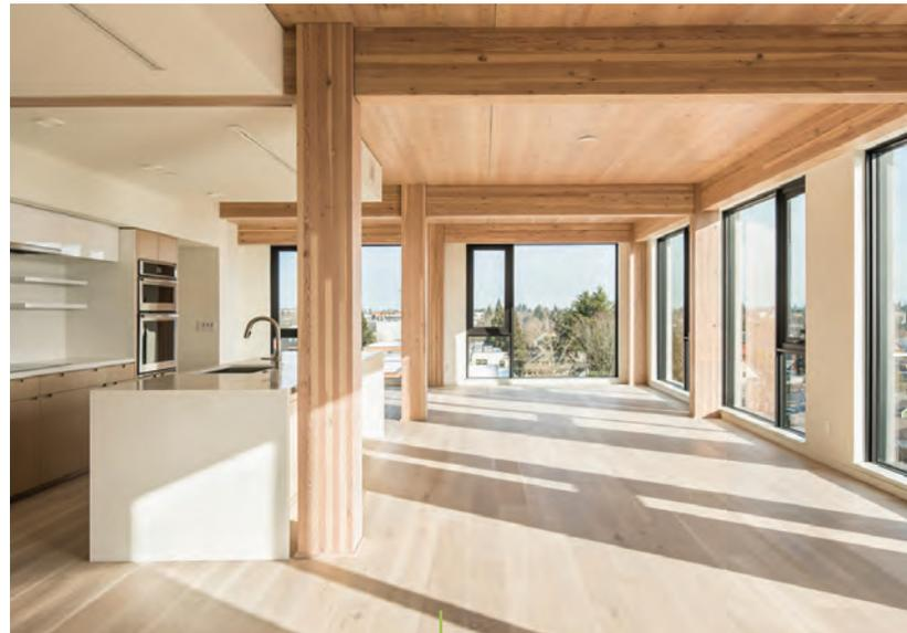
Char calculations can be used to demonstrate fire-resistance ratings.<sup>3</sup> This method accounts for mass timber's ability to form a char zone when subjected to fire, which insulates the remaining wood cross-section, allowing it to retain structural capacity. Carbon12, Path Architecture, Munzing Structural Engineering, Kaiser Group
