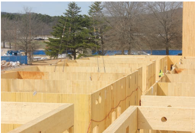
Interior partitions in a four-story CLT hotel
