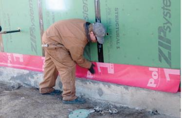
• **Geotextile membranes** come in a variety of configurations to protect various parts of a structure. Under-slab sheets include 8.5 mils of high-strength crosslaminated polyethylene backing topped with a 69-mil-thick layer of barrier sealant integrated into a high strength non-woven geotextile fabric. Peel-and-stick barriers, which come in large sheets or a variety of roll widths, consist of a 4-mil-high density polyethylene film bonded to 36 mils of sealant.<sup>7</sup>
