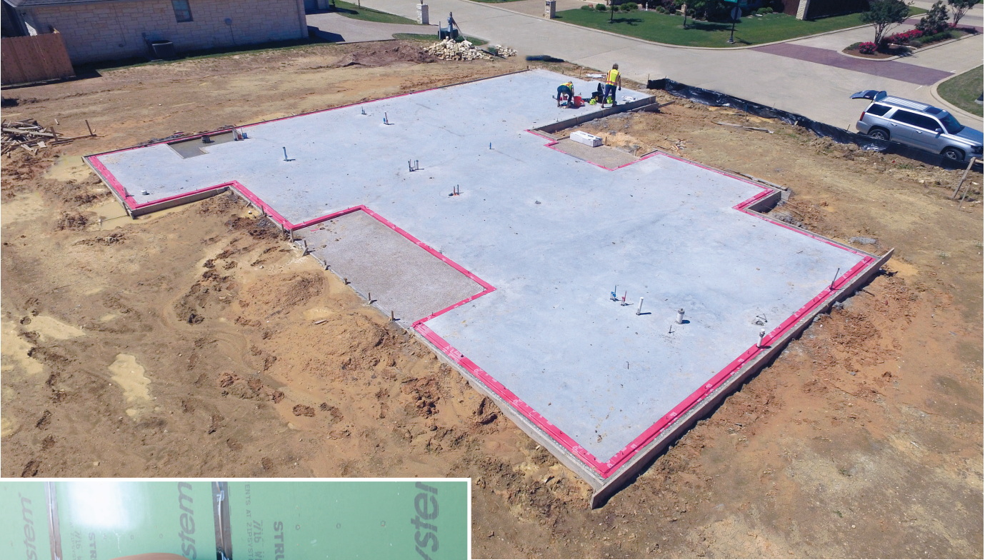
Peel-and-stick flashing moisture/termite barrier (left); undersill moisture/termite barrier (above)
