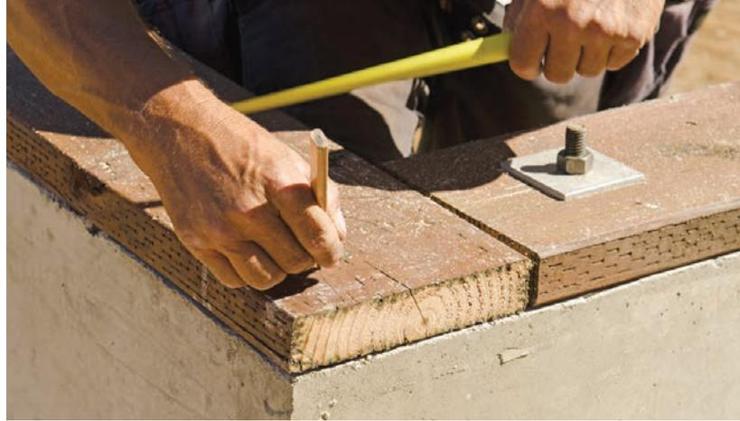
Pressure-preservative-treated wood used as sill plates. The IBC requires that surface treatments be applied to end cuts and holes.
