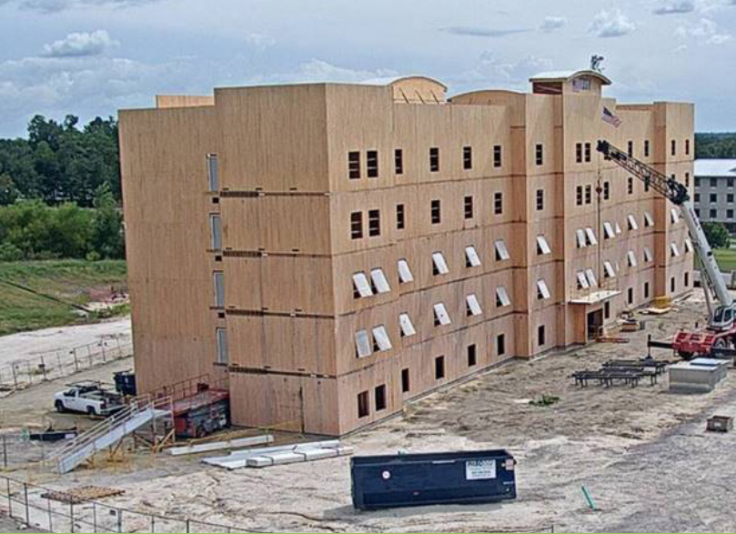
When it was built, Candlewood Suites at Fort Jackson, South Carolina was the largest CLT project in the Eastern U.S., and one of the 10 largest in the country.
