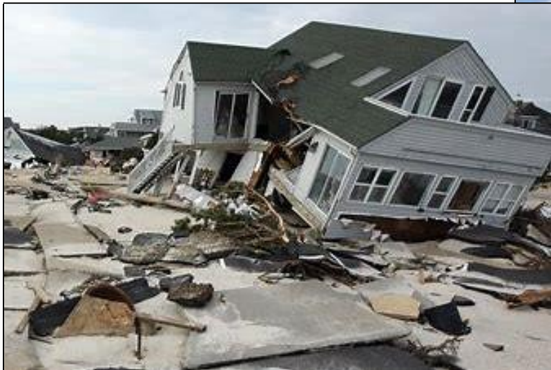
Possible Soft Story (Not enough shear walls across front)
