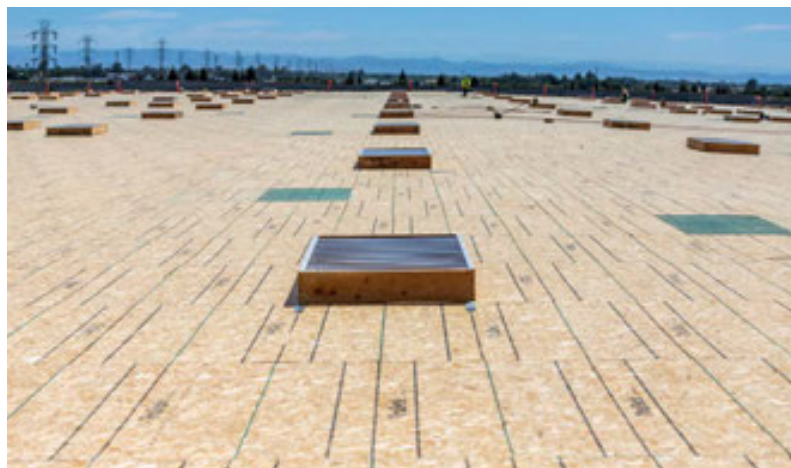
Installation of beams prior to panels in all-wood roof system (left); panelized wood roof with skylight fall protection (right)
