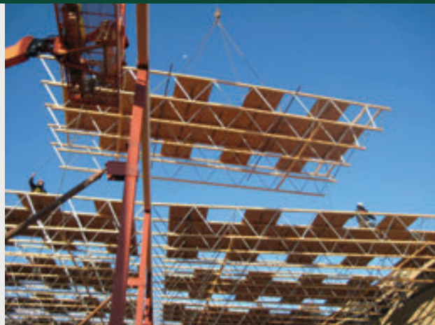
Photo: Mandere Construction
