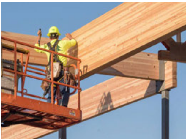
Installation of beams prior to panels in all-wood roof system (left); panelized wood roof with skylight fall protection (right)
