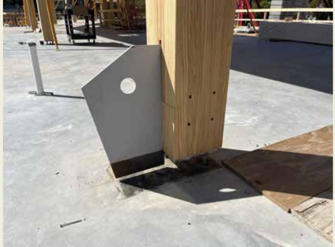
Example of custom hardware with construction tolerance.
