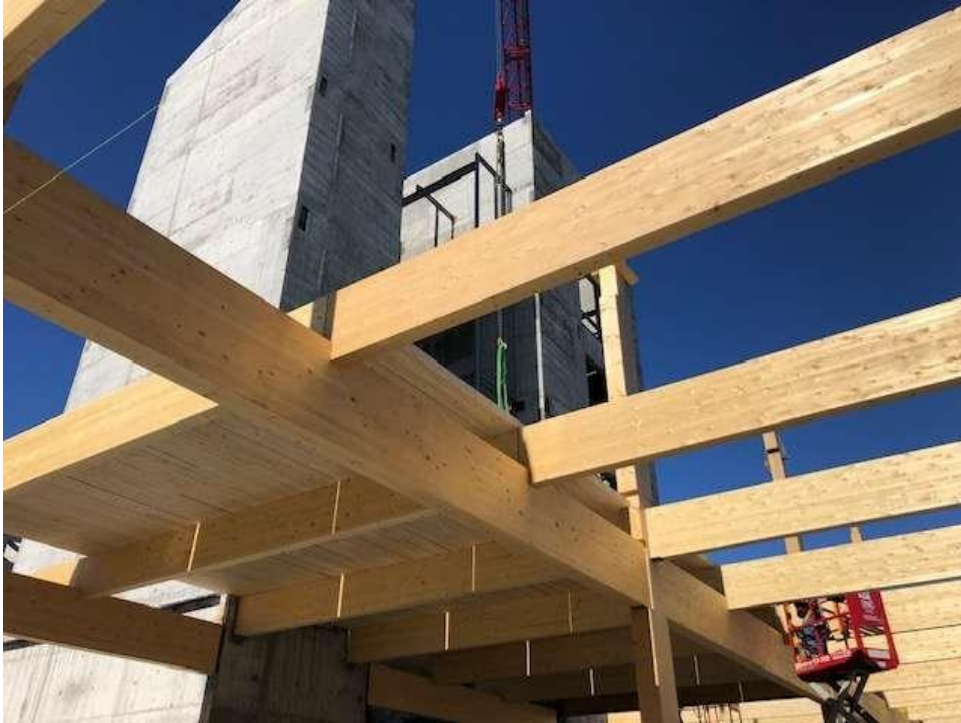
Simple Bearing Connections
