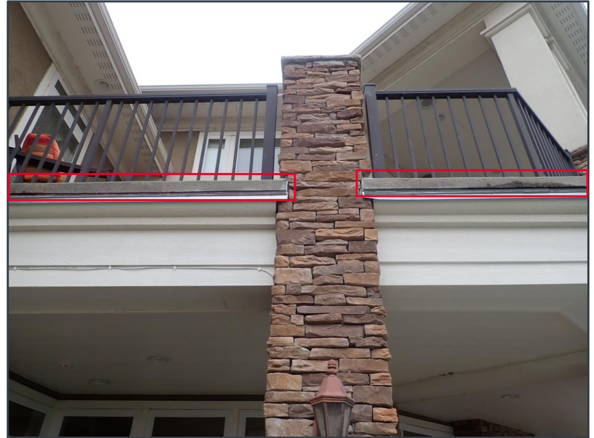
Concrete topping slab above OSB substrate and wood joists - WPM
