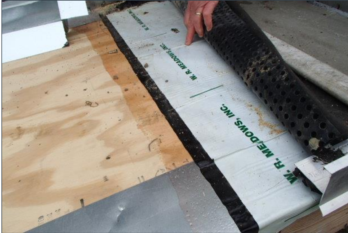
Pre-construction testing and inspection of deck waterproofing system field mockup - WPM
