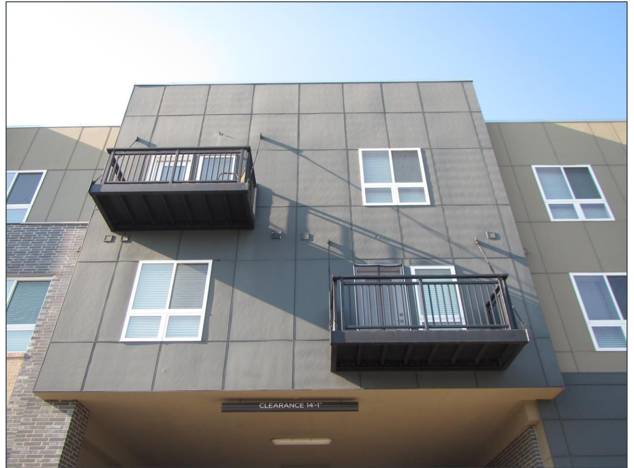
Prefabricated steel balcony bolted onto rainscreen building façade - WPM
