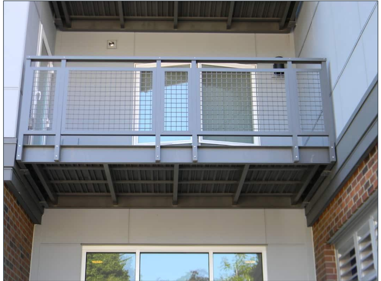
Prefabricated aluminum balcony – WPM
