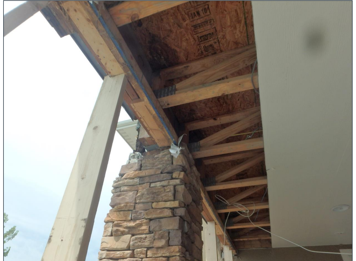
Wood joists with Oriented Strand Board (OSB) layers above - WPM
