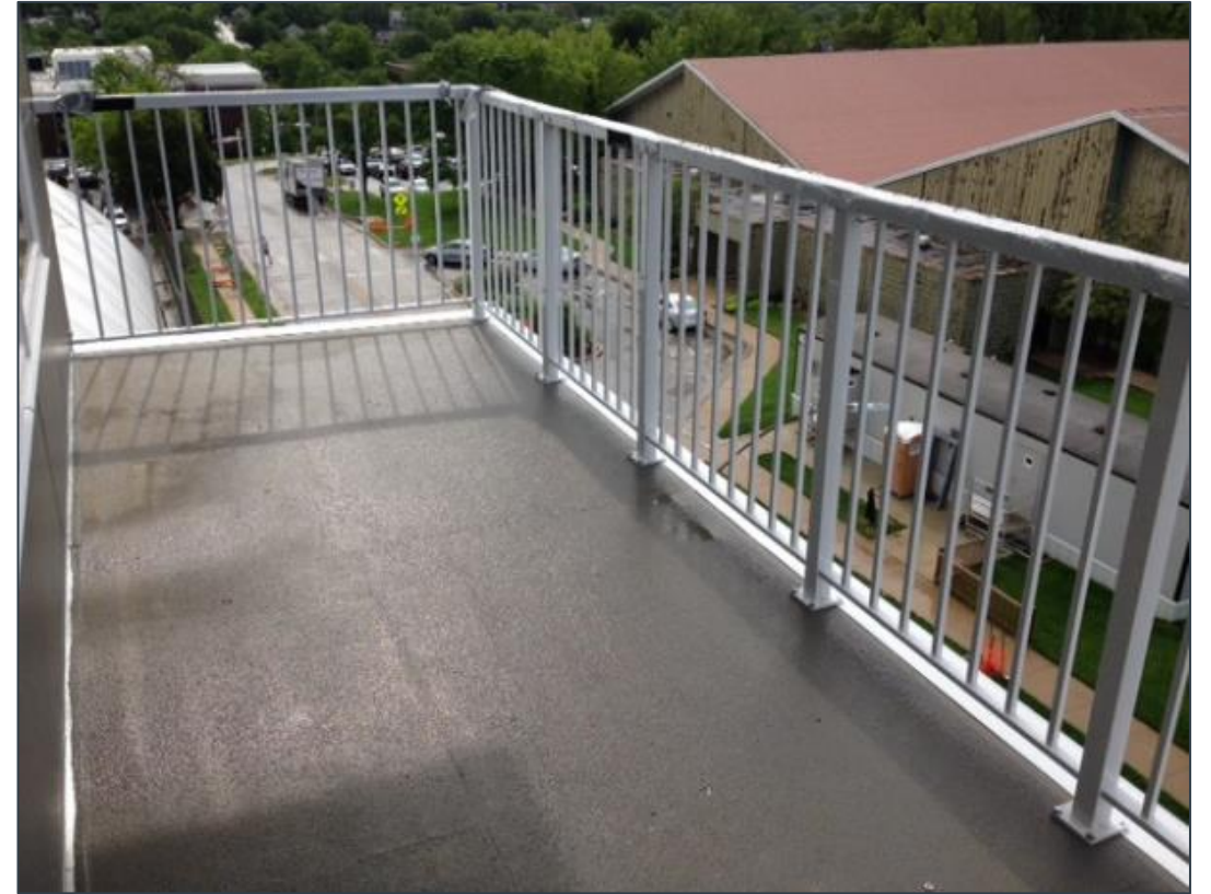
Pre-construction testing and inspection of handrail connection field mockup - WPM
