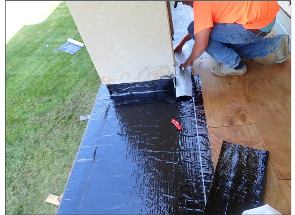
Sheet waterproofing membrane system fitted around existing balcony column and over plywood decking - WPM
