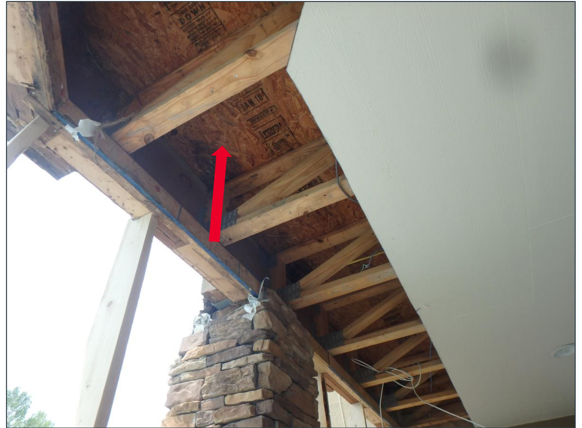
OSB sheets set above wooden structural beams and joists - WPM
