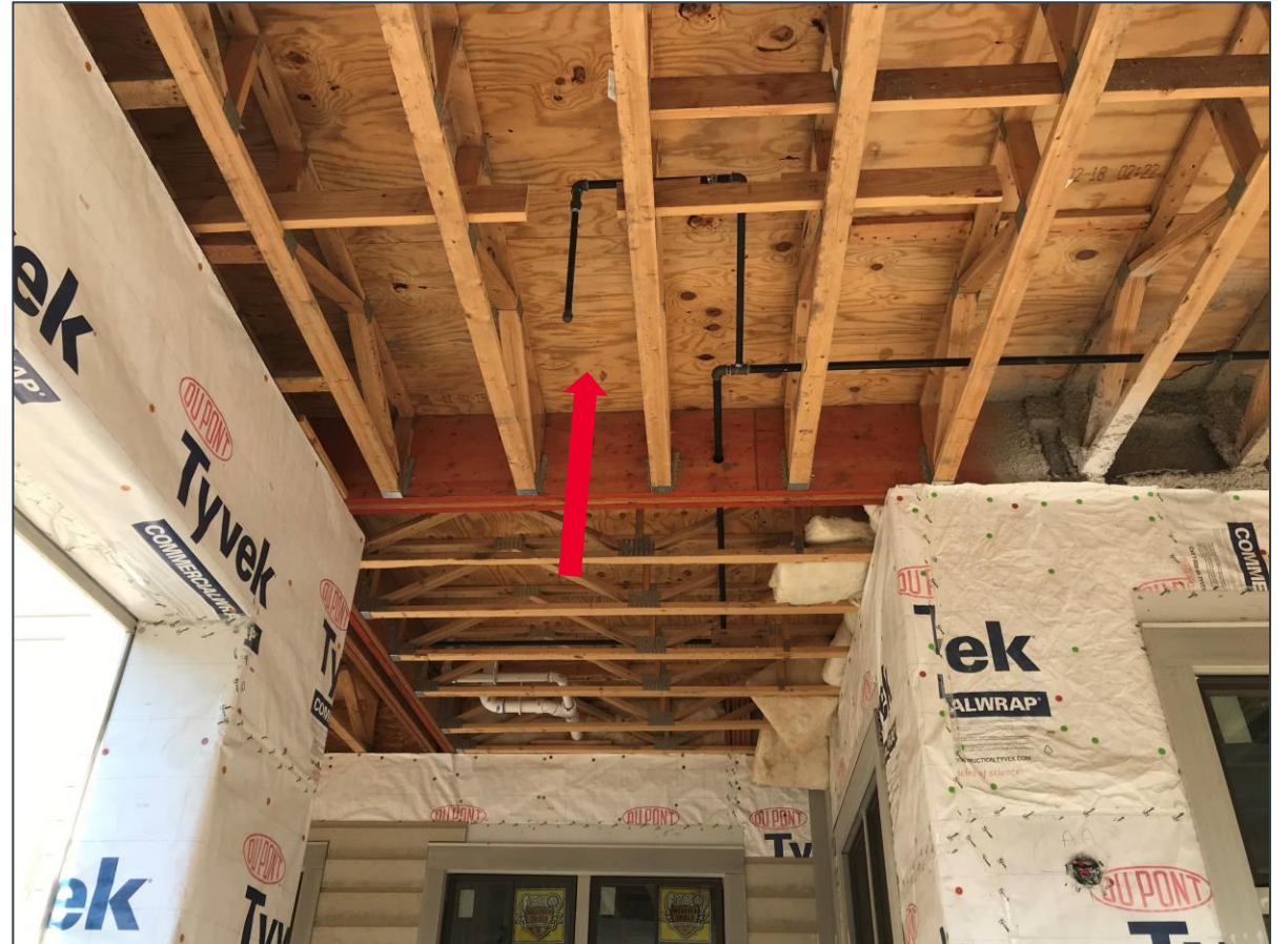
Plywood sheets set above wooden structural beams and joists - WPM
