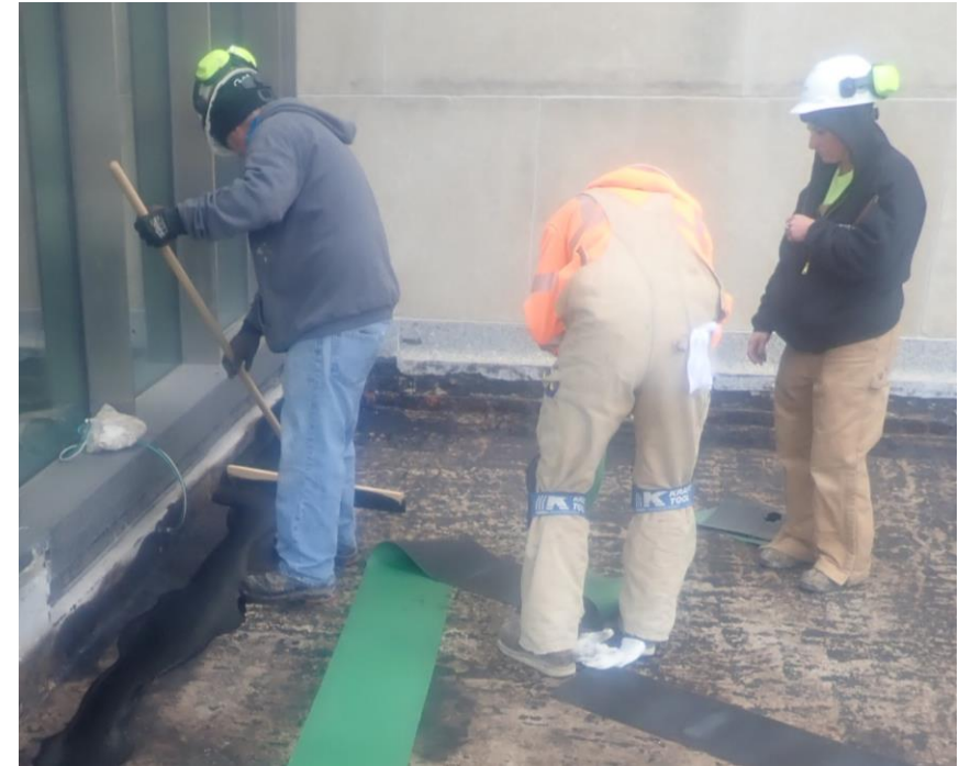
Application of hot rubberized asphalt membrane
