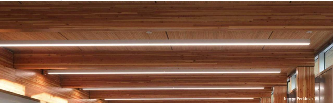
Type IV construction permits exposed heavy/mass timber elements of min. sizes.
