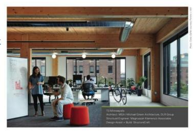
The growing availability and code acceptance of mass timber-i.e., large solid wood panel products such as crosslaminated timber (CLT) and nail-laminated timber (NLT)for floor, wall and roof construction has given designers a low-carbon alternative to steel, concrete, and masonry for many applications. However, the use of mass timber in multi-family and commercial buildings presents unique acoustic challenges.
