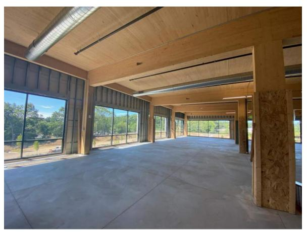
Connection FRR and beam reactions could impact required beam/column sizes
