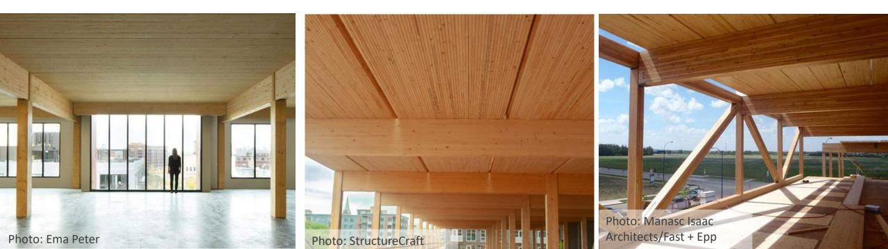
Cross-Laminated Timber (CLT) Solid sawn laminations
