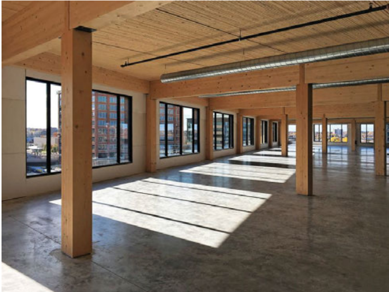
T3 Minneapolis Minneapolis, MN Image Credit: Blaine Brownell
