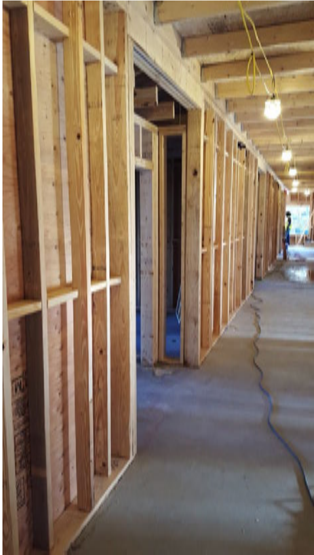
Light-Frame Wood Photo: WoodWorks
