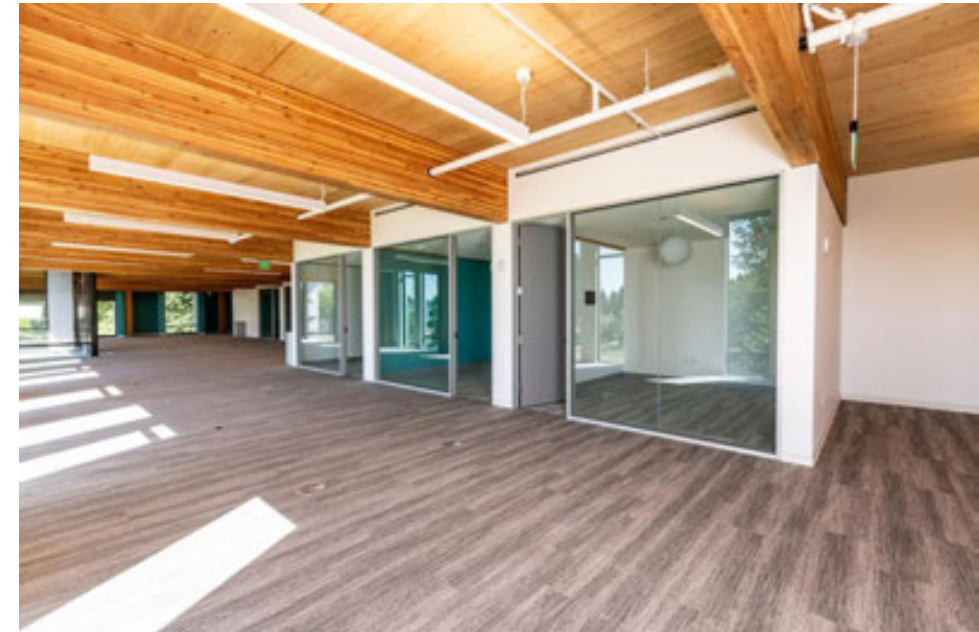
First Tech Credit Union, Hillsboro, OR 12x32 Grid, One-Way Beams 5-ply (5.5") CLT Image: Swinerton
