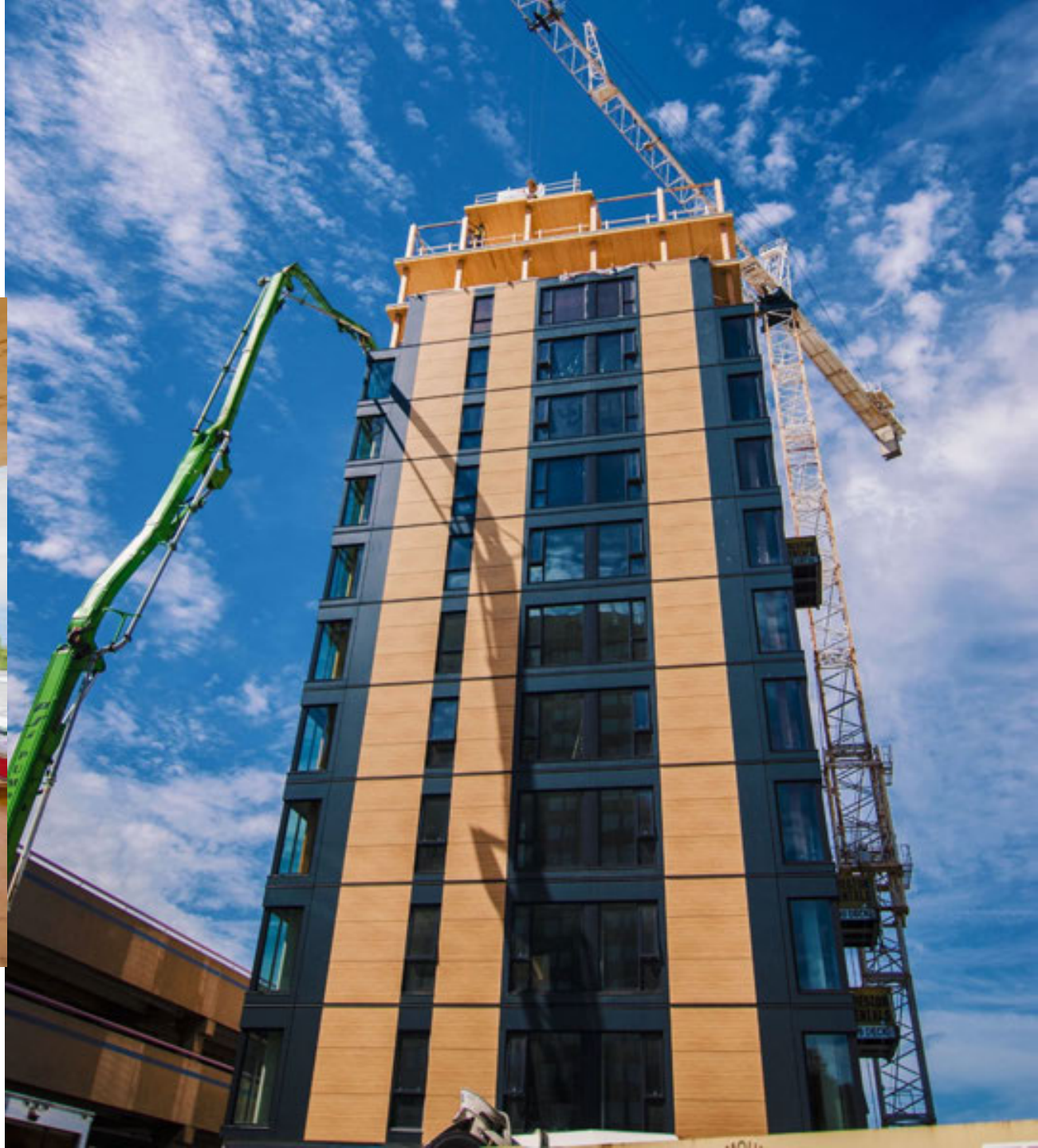
Brock Commons Vancouver, BC Images: Acton Ostry Architects
