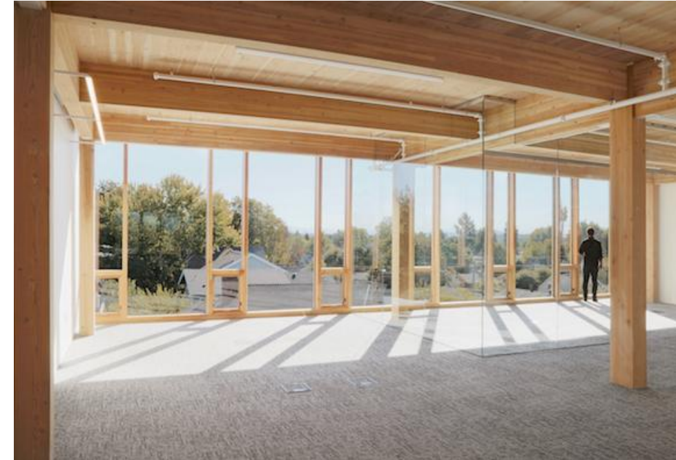
Albina Yard, Portland, OR 20x20 Grid, 1 purlin per bay 3-ply CLT Image: Lever Architecture
