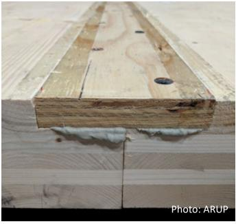
Several MT fire tested assemblies have successfully been completed w/o adhesives/sealants at abutting panel edges
