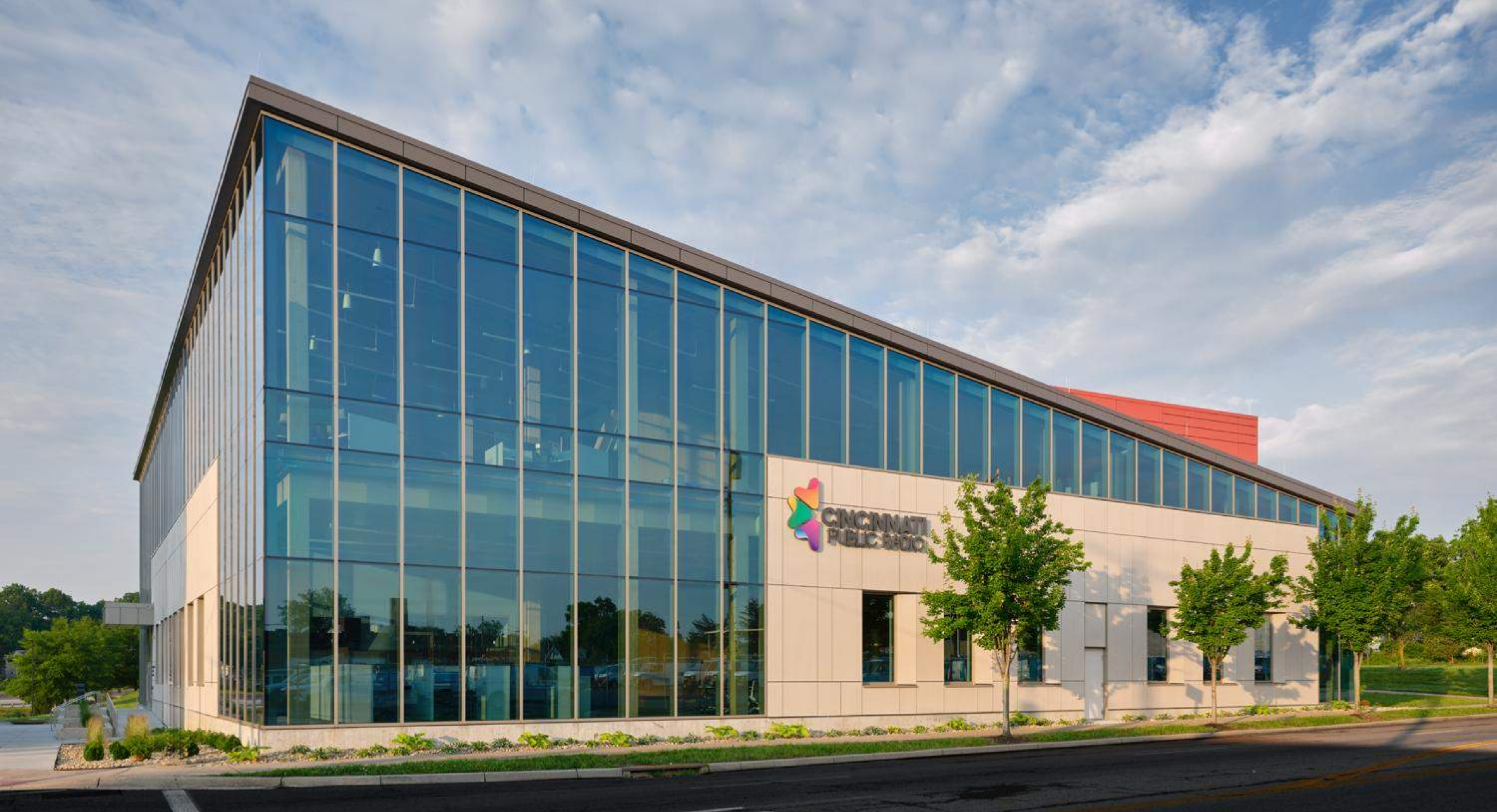
Exterior – North view
