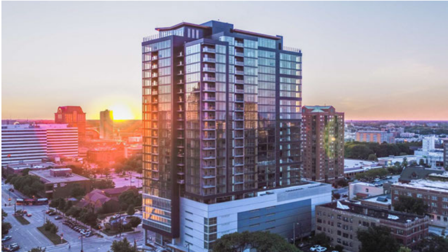
Ascent – Photo: CD Smith Construction
