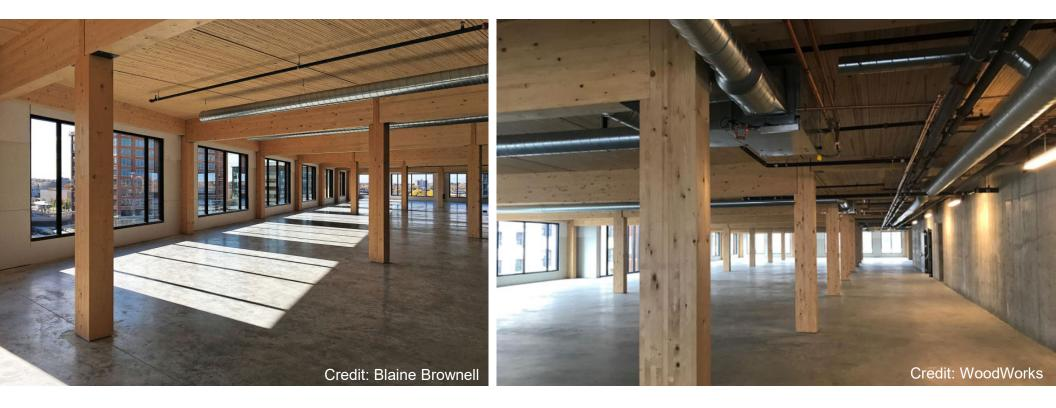
Grid impact: Relies on one-way beam layout. Columns/beams spaced at panel span limits in one direction.
