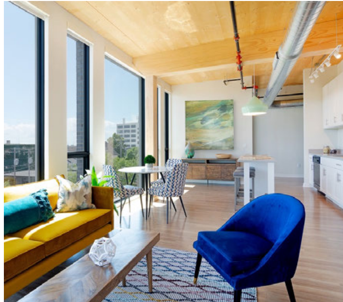
MT Floors & Roofs on Post & Beam Framing
