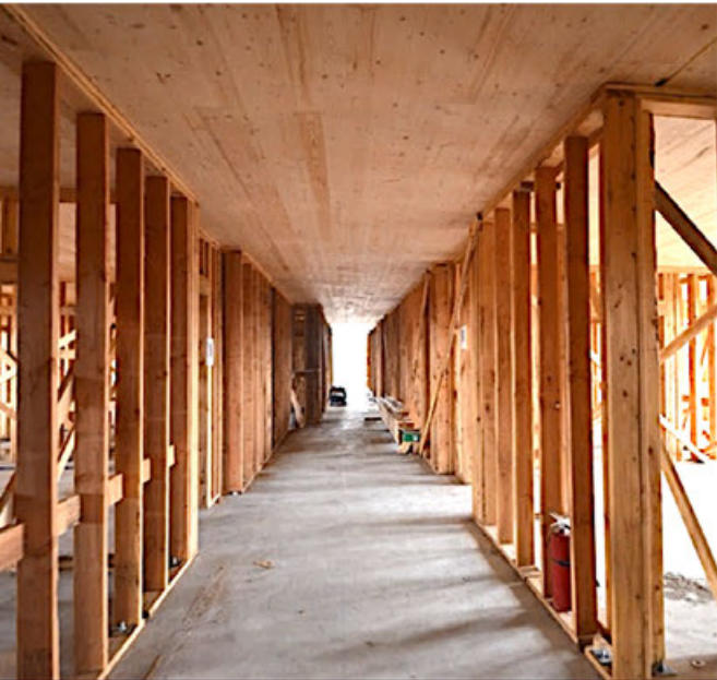
MT Floors & Roofs on LWF Bearing Walls
