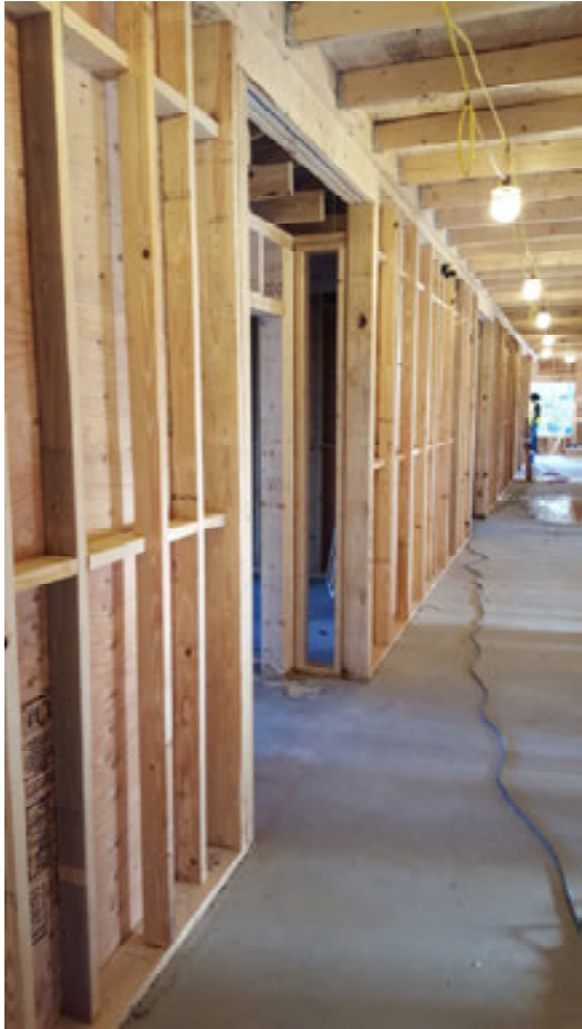
Light Wood-Frame Photo: WoodWorks
