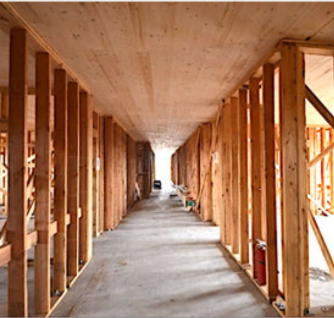
MT Floors & Roofs on LWF Bearing Walls
