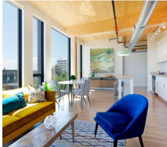
MT Floors & Roofs on Post & Beam Framing
