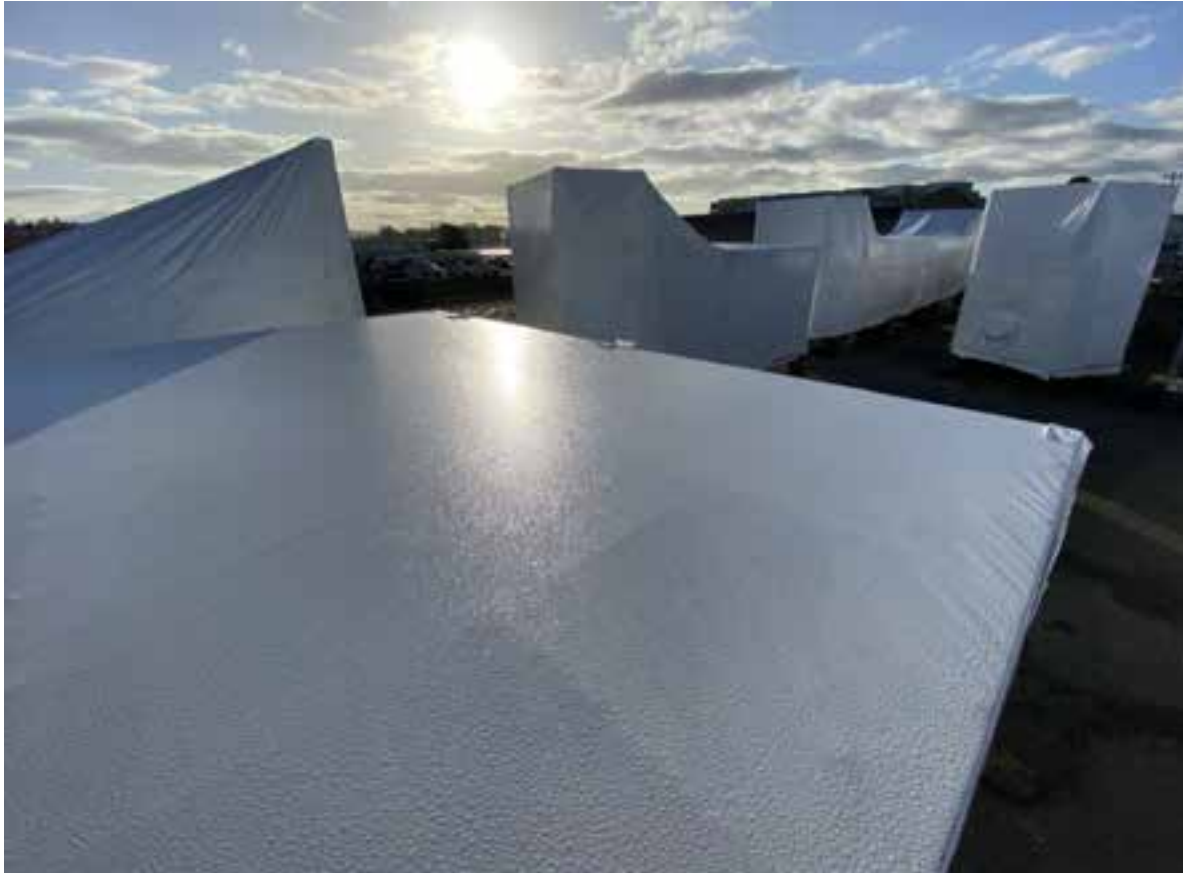
Morning condensation on shrink wrap protecting roof of mods
