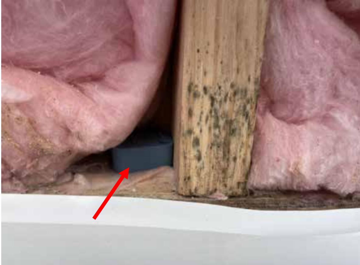
Temperature/humidity sensor installation
