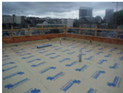
Self-adhered membrane over wood deck
