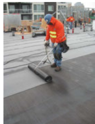
Torch-applied modified bitumen membrane over concrete deck
