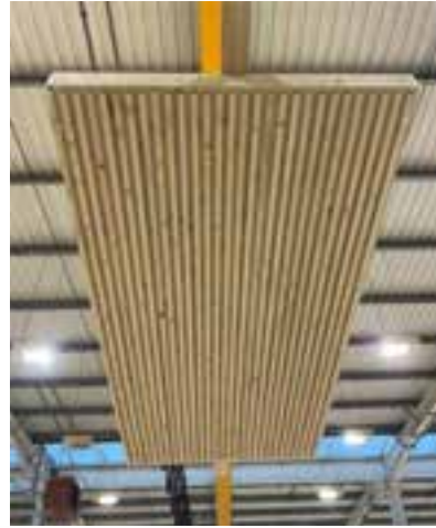
NLT Ceiling Panels (using beech nails)
