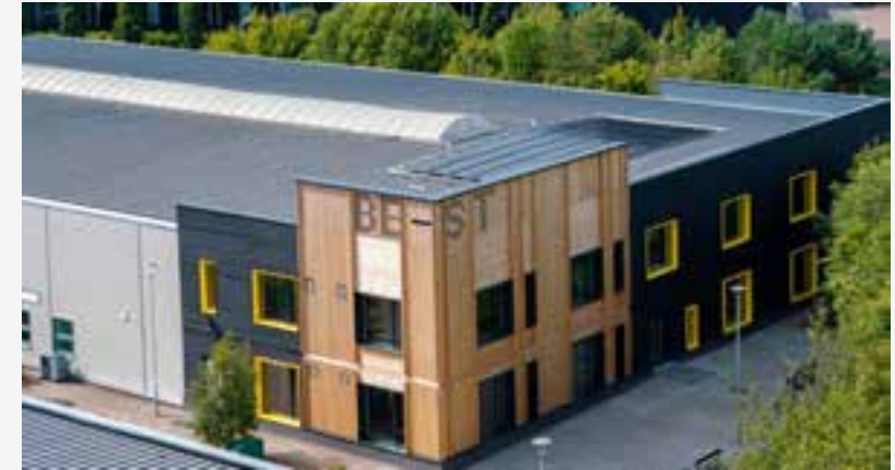
SNRC Retrofit – BE-ST
