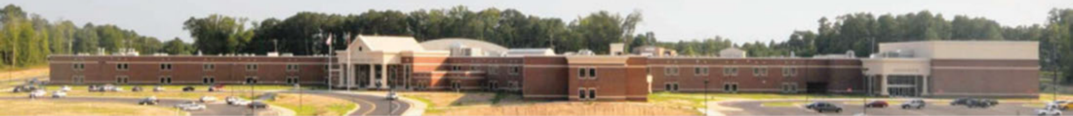
El Dorado High School / CADM Architecture / Engineering Consultants / Photo Dennis Ivy
