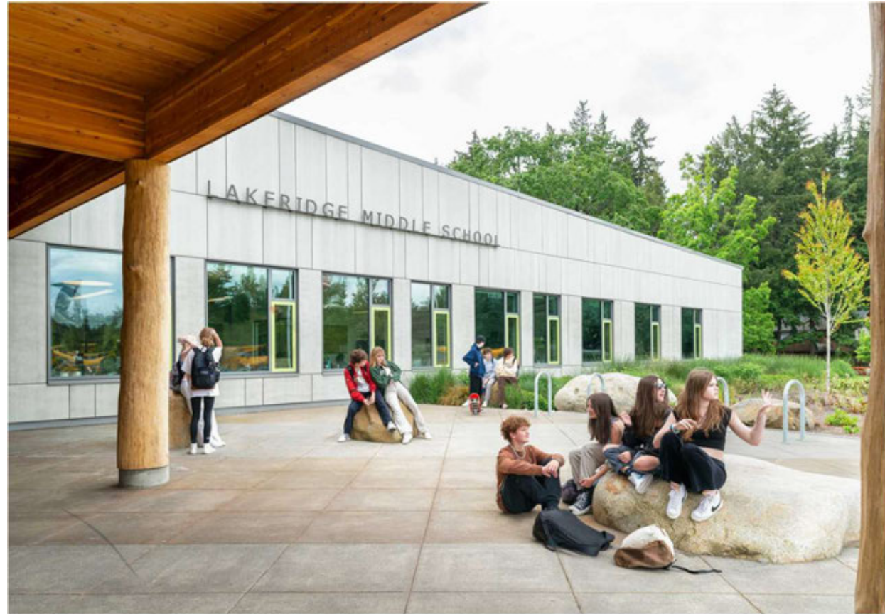
Lakeridge Middle School / Mahlum Architects / KPFF / Photo Arthur Ross
