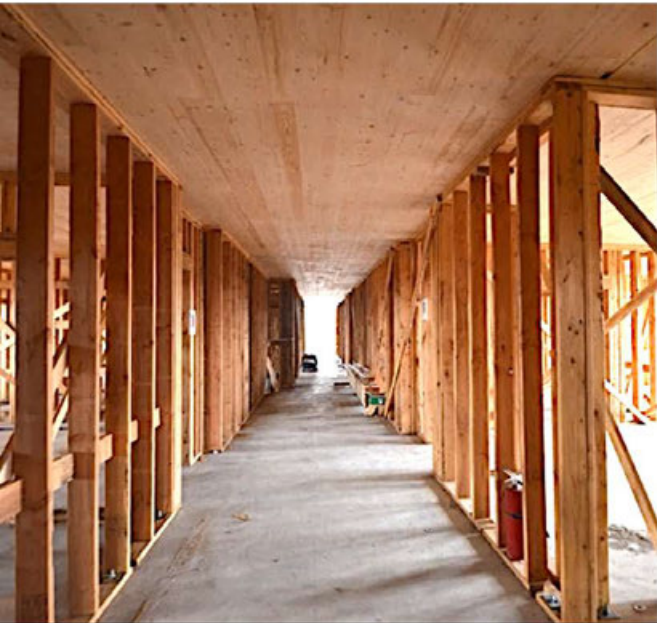
MT Floors & Roofs on LWF Bearing Walls
