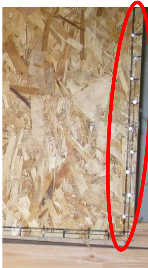
Nailing not staggered
