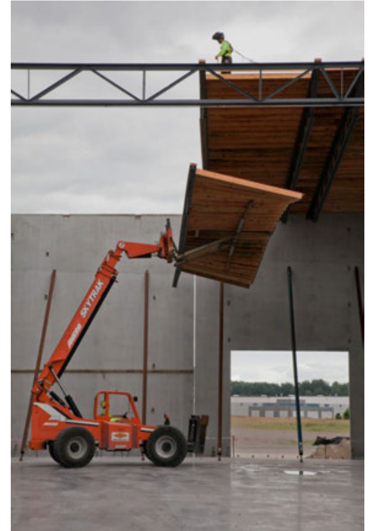
Photo: Panelized Structures
