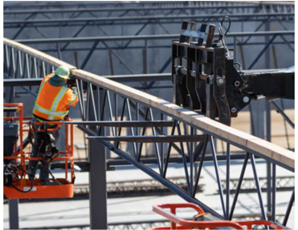
Photos: Panelized Structures
