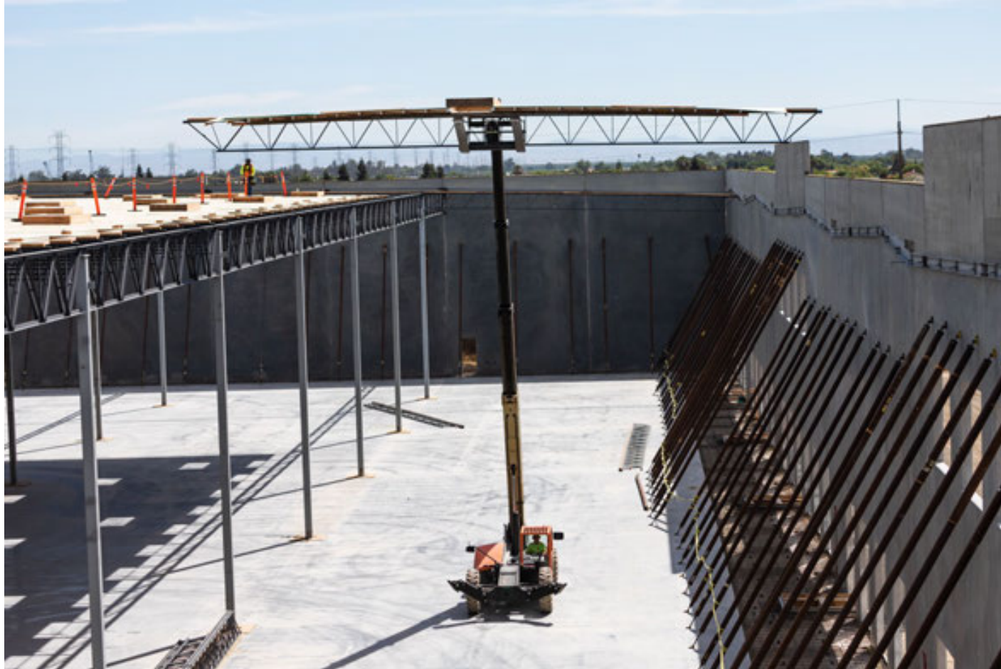
Photo: Panelized Structures
