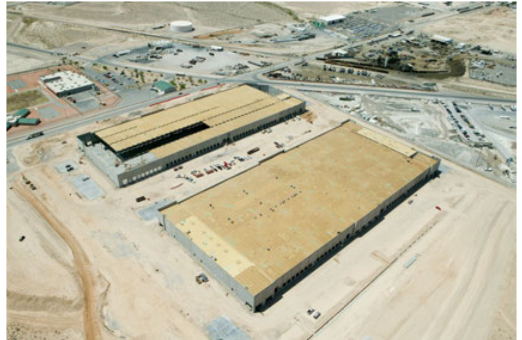
Photo: Panelized Structures
