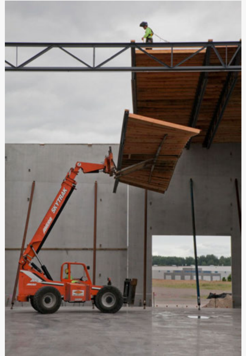
Photo: Panelized Structures
