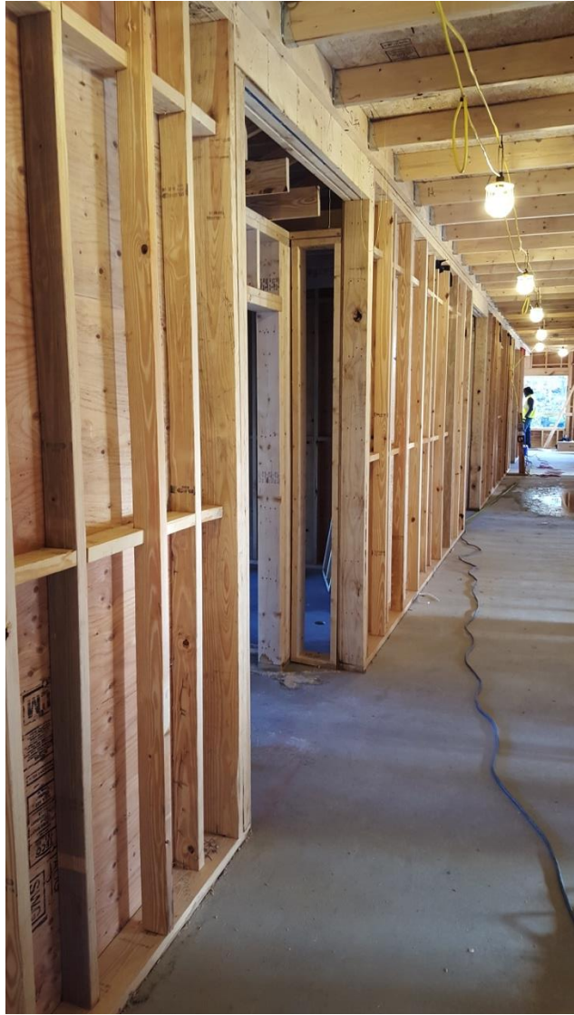
Light-Frame Wood Photo: WoodWorks
