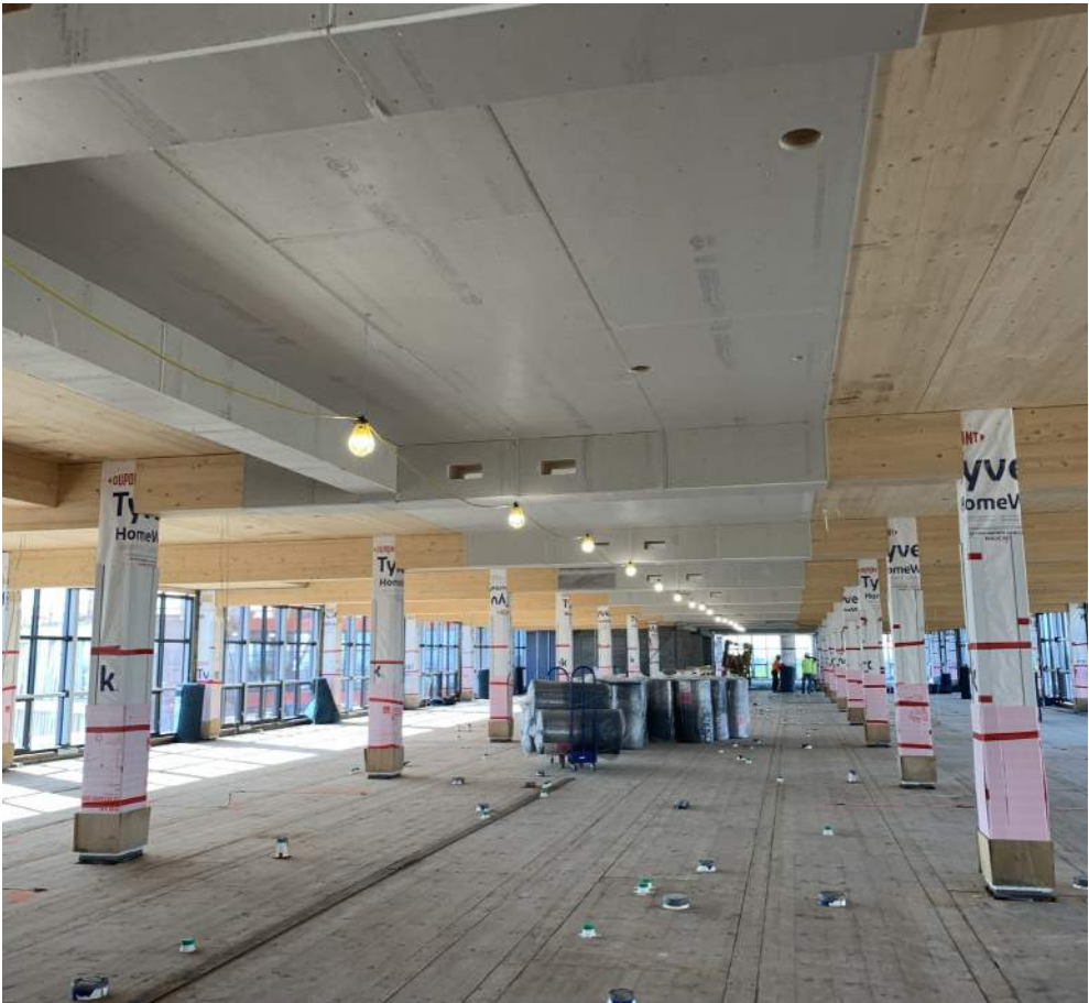
ADDED CORRIDOR DRYWALL INSTALLED PRIOR TO ACOUSTIC MAT AND TOPPING SLAB
