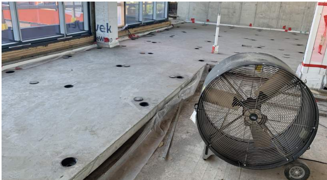
FLOATING SLAB INSTALLATION IN PROGRESS
