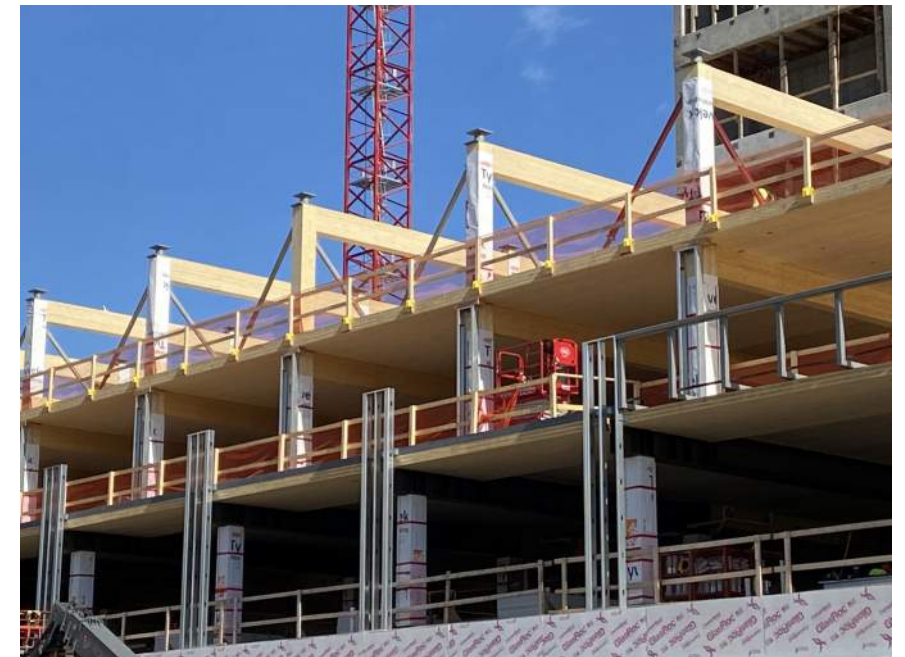
TEMPORARY PROTECTION OF TIMBER IN PLACE
