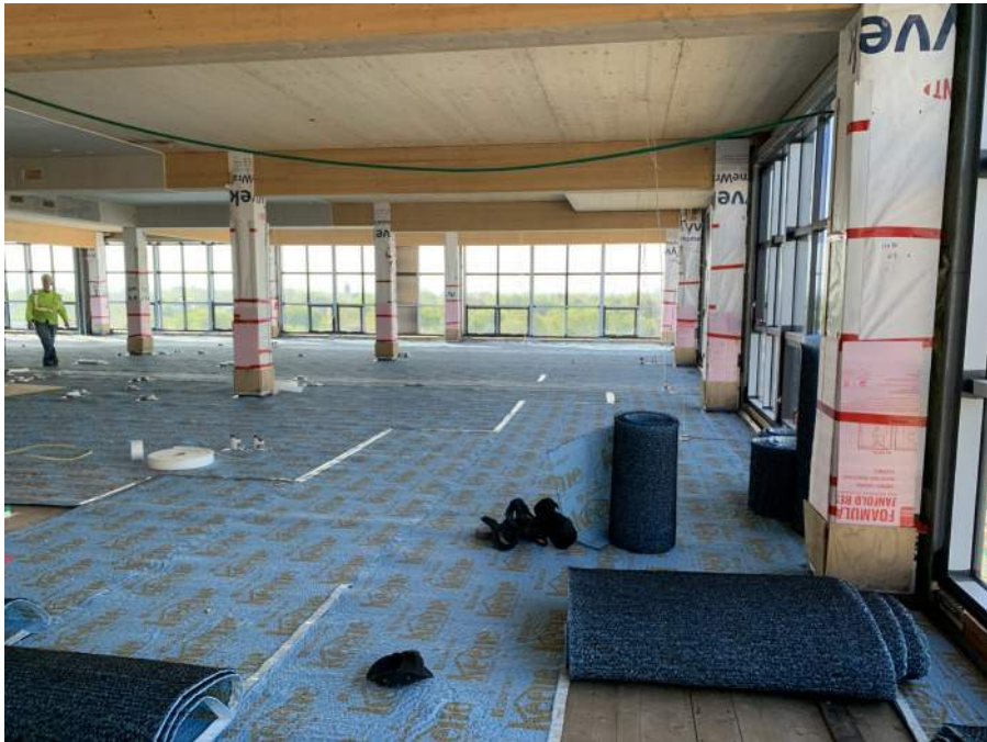
ACOUSTIC MAT INSTALLATION IN PROGRESS
