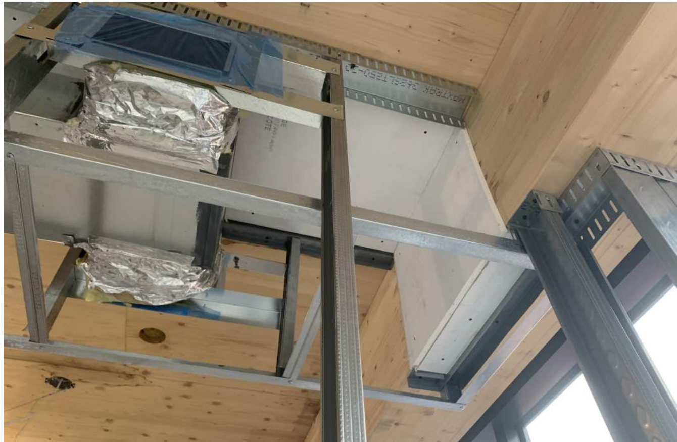
DRYWALL ENCAPSULATION AT DUCT SOFFIT
