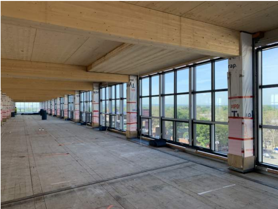
CLT DECK PREPPED FOR ACOUSTIC MAT LAYOUT
