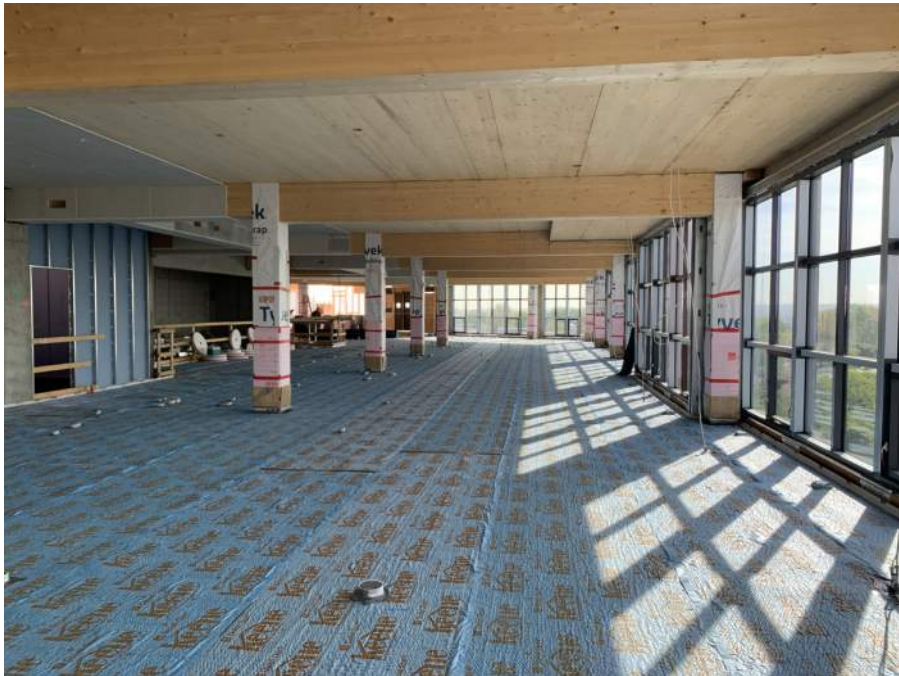
ACOUSTIC MAT INSTALLATION COMPLETE AND READY FOR TOPPING SLAB
