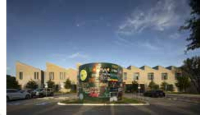
Water Collection Tank
