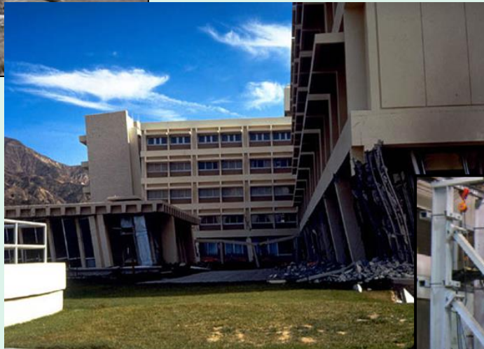
Seismic (soft story)
