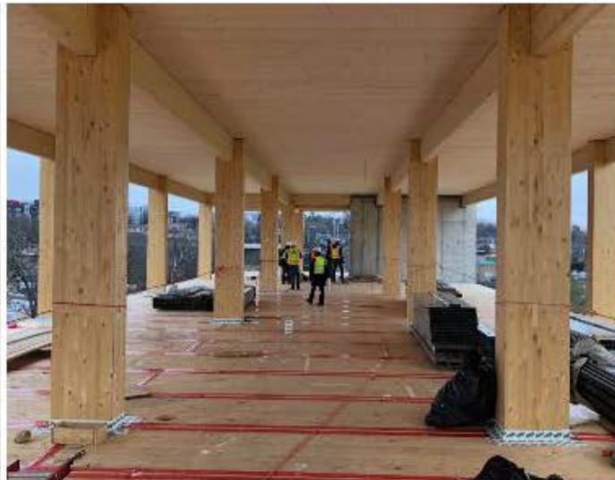
column & beams & panel
