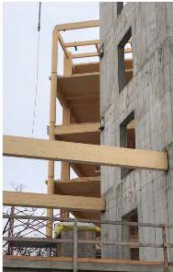
Connection between beams & core
