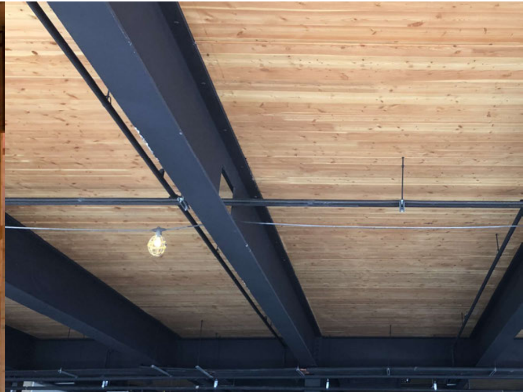
Hybrid: Steel framing
