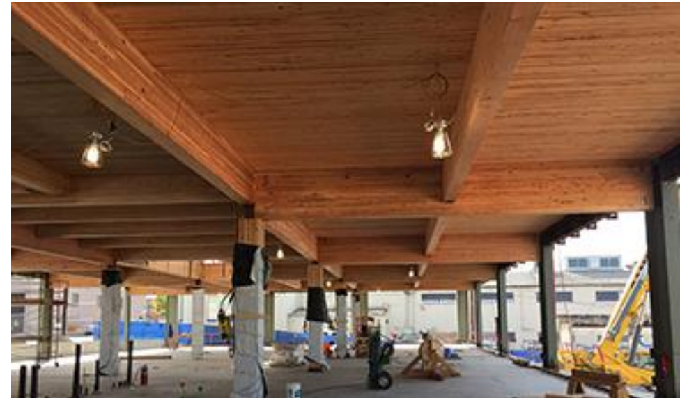
Clay Creative, Portland, OR 30x30 Grid, 1 purlin per bay 2x6 NLT Image: Mackenzie
