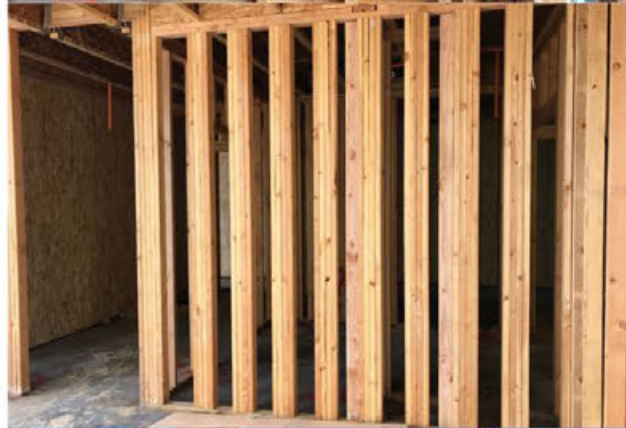
2X4 Framed Interior Bearing Wall Stud Packs
