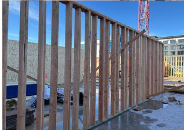
Staggered Stud on Single Plate
