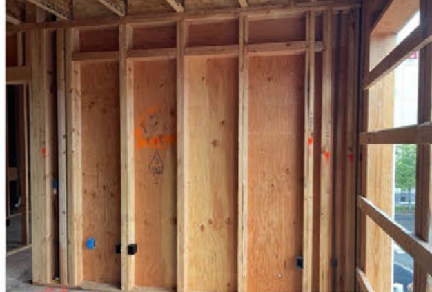
2X6 Stacked Framed Interior Bearing Wall
