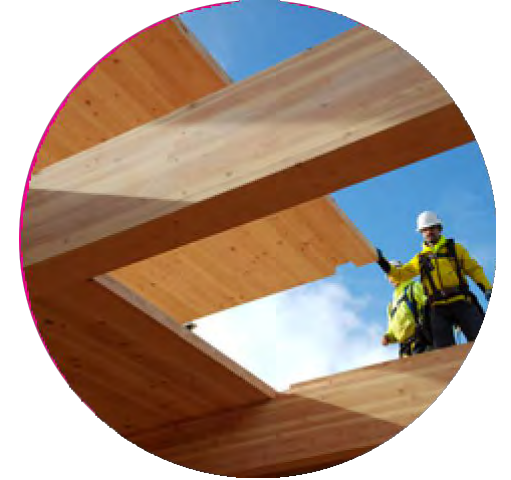
CLT panels are used to construct mass timber building at Ponce City Market in Atlanta
