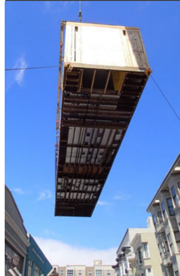
Volumetric Modular (Light-frame)
