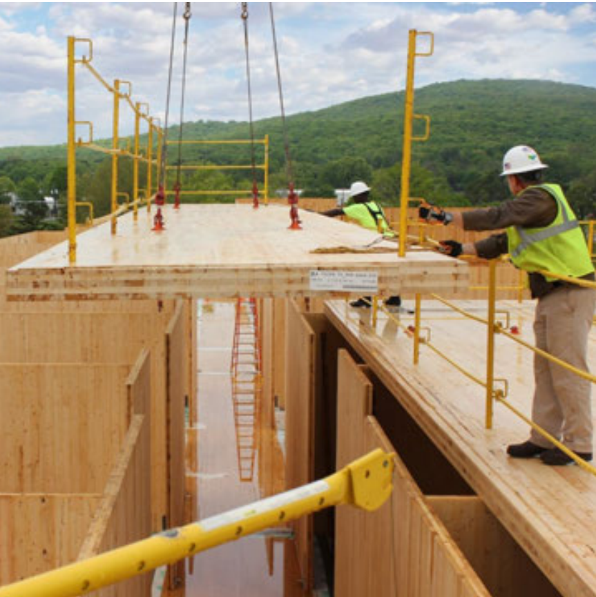
Developer, Asset Manager, Design Builder: Lendlease Locations: Redstone Arsenal, Huntsville, Alabama
