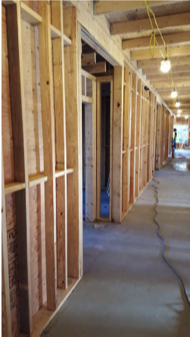
Light-Frame Wood Photo: WoodWorks
