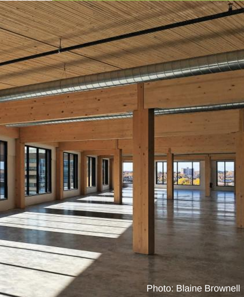
Post and Beam
