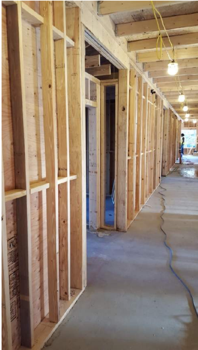
Light-Frame Wood Photo: WoodWorks
