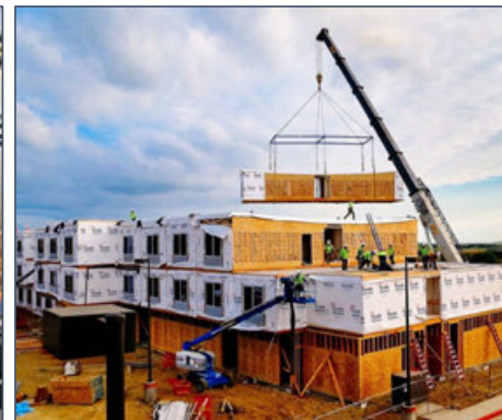
Modules Are Stacked and Assembled At The Construction Site
