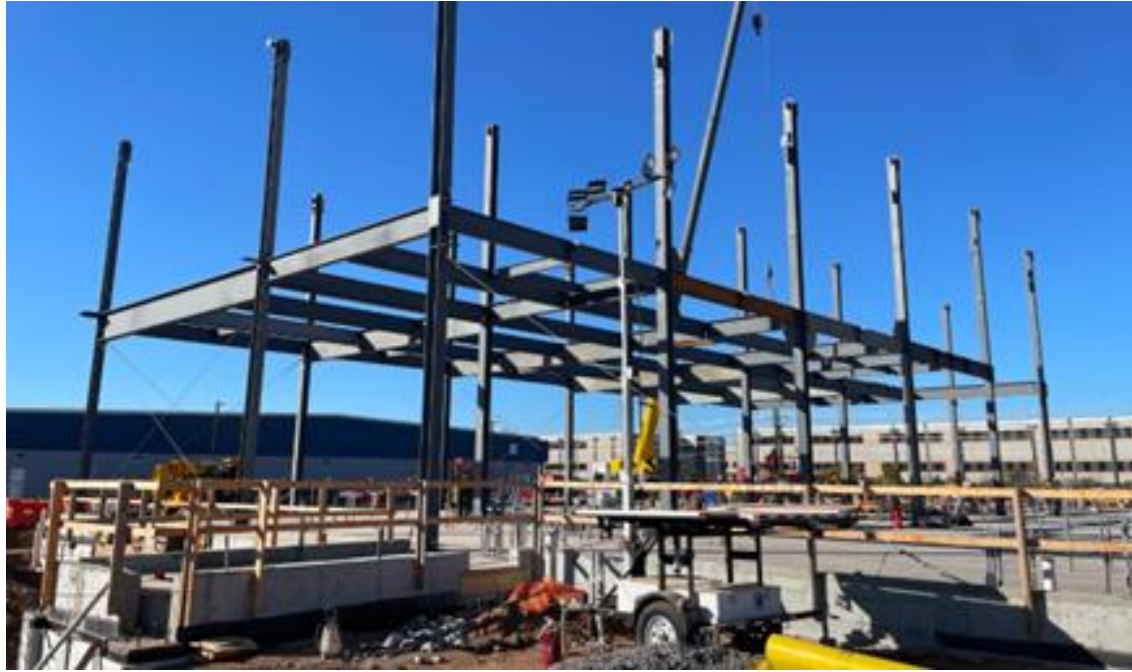
Erection of Steel Frame
