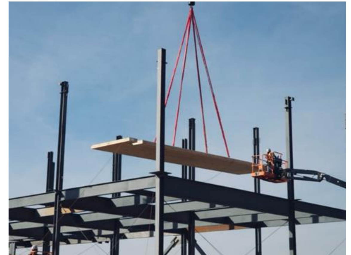
Securing of CLT by Steel Erectors
