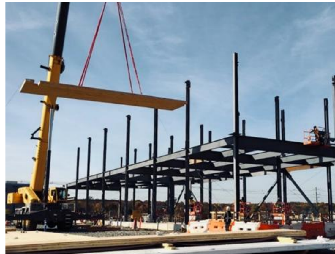
Erection of CLT Panel
