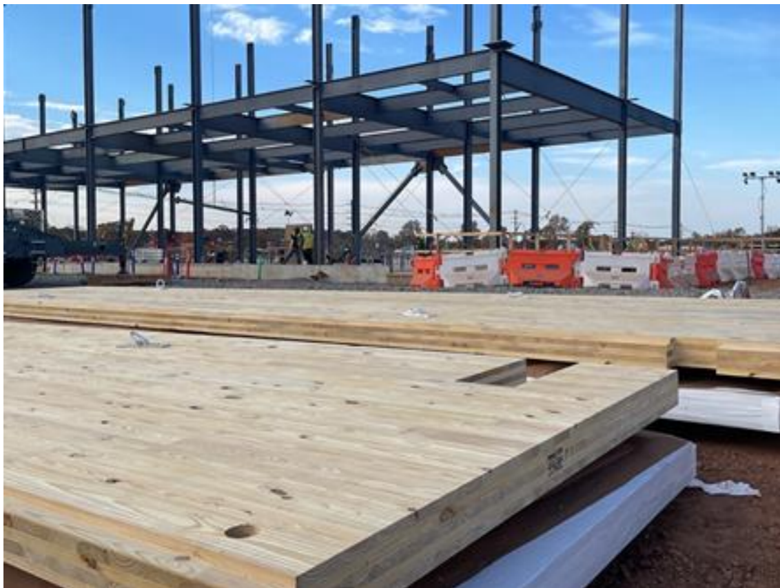
CLT Prep and Inspection
