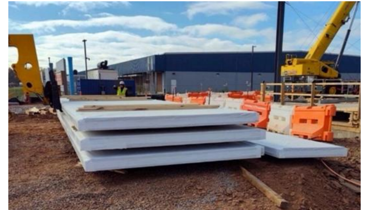
Storage of CLT Panels
